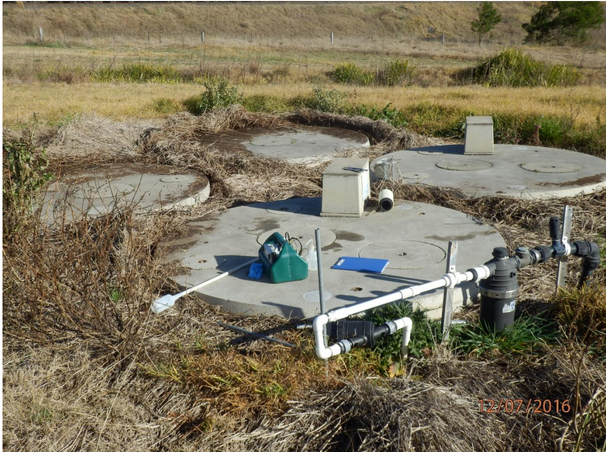
Attachment B, Figure 1 Econocycle wastewater system, foreground pipes to irrigation area
