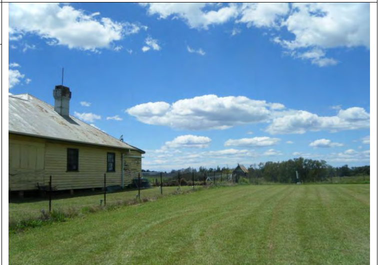
Photo 6 – North of the stockpile area (255 m)
