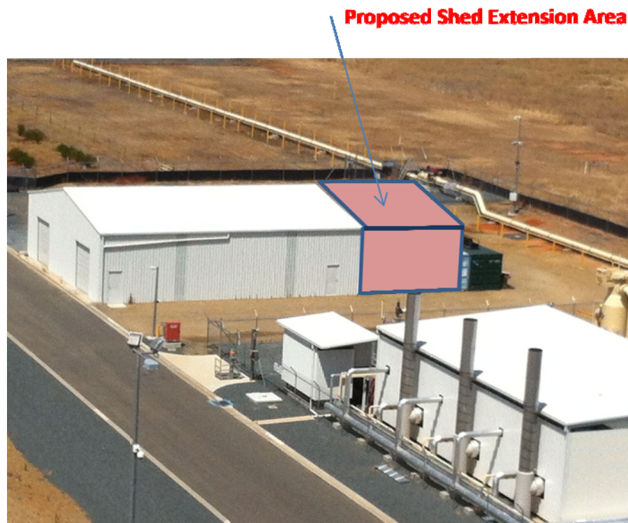
Figure 1. Existing Storage Shed looking South West & shipping containers being used for temporary storage
