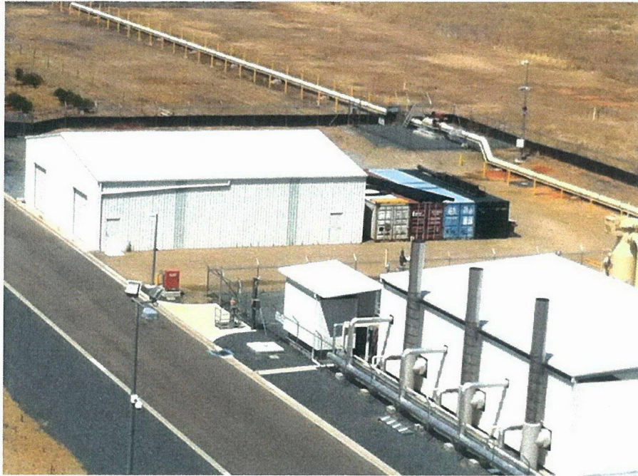
Figure 1. Existing Storage Shed looking South West & shipping containers being used for temporary storage
