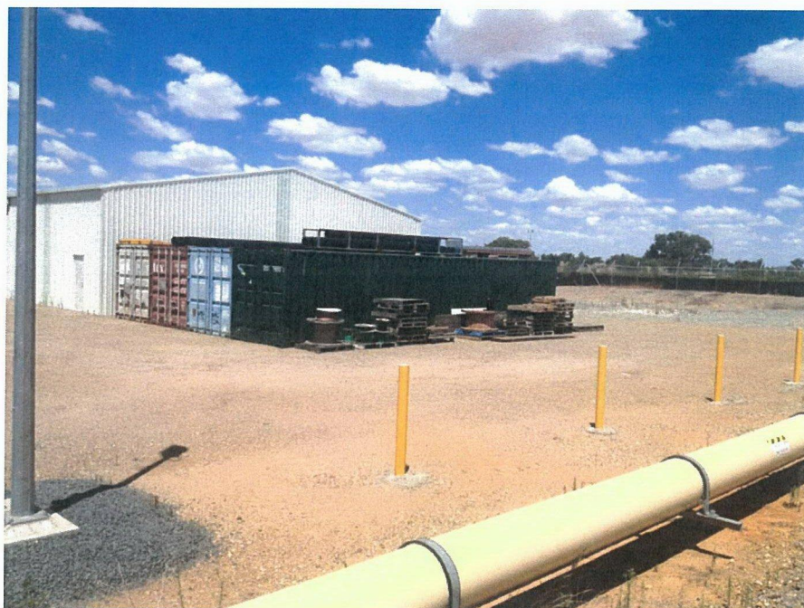
Figure 3. Existing Storage Shed showing proposed extension area where shipping containers are currently stored and the gas pipeline in foreground.
