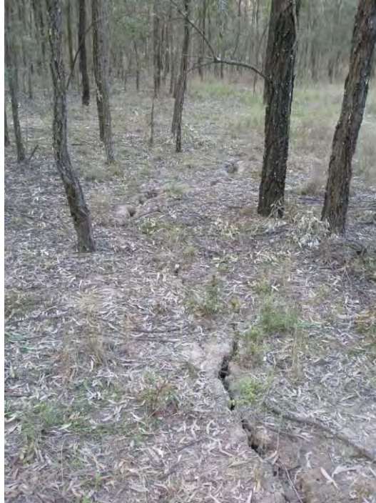
Plate 3 – Soil Cracking Observed at Wambo
