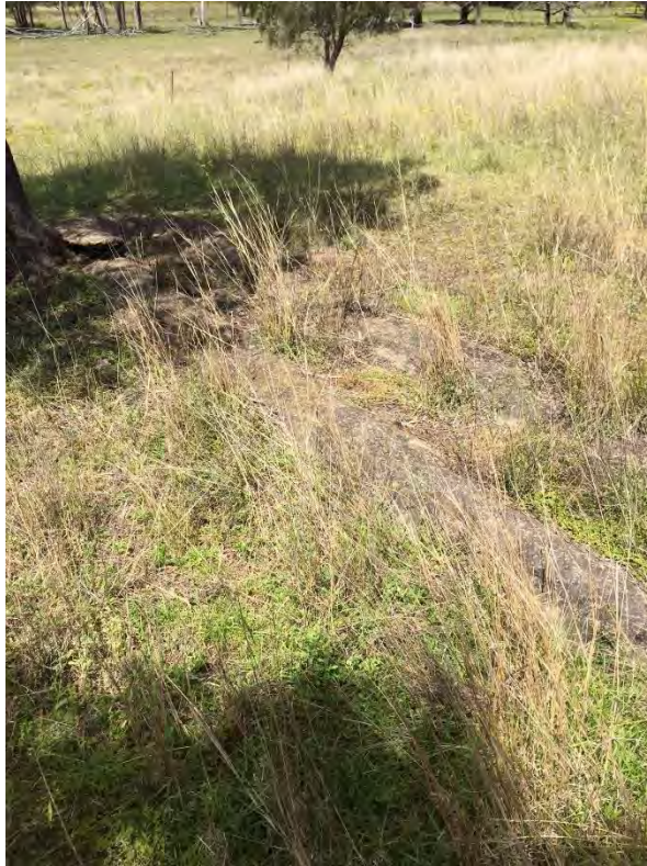
Photograph 11 – Concrete dish drain/spoon drain against eastern fence line. Potentially former trough or feeding structure.
