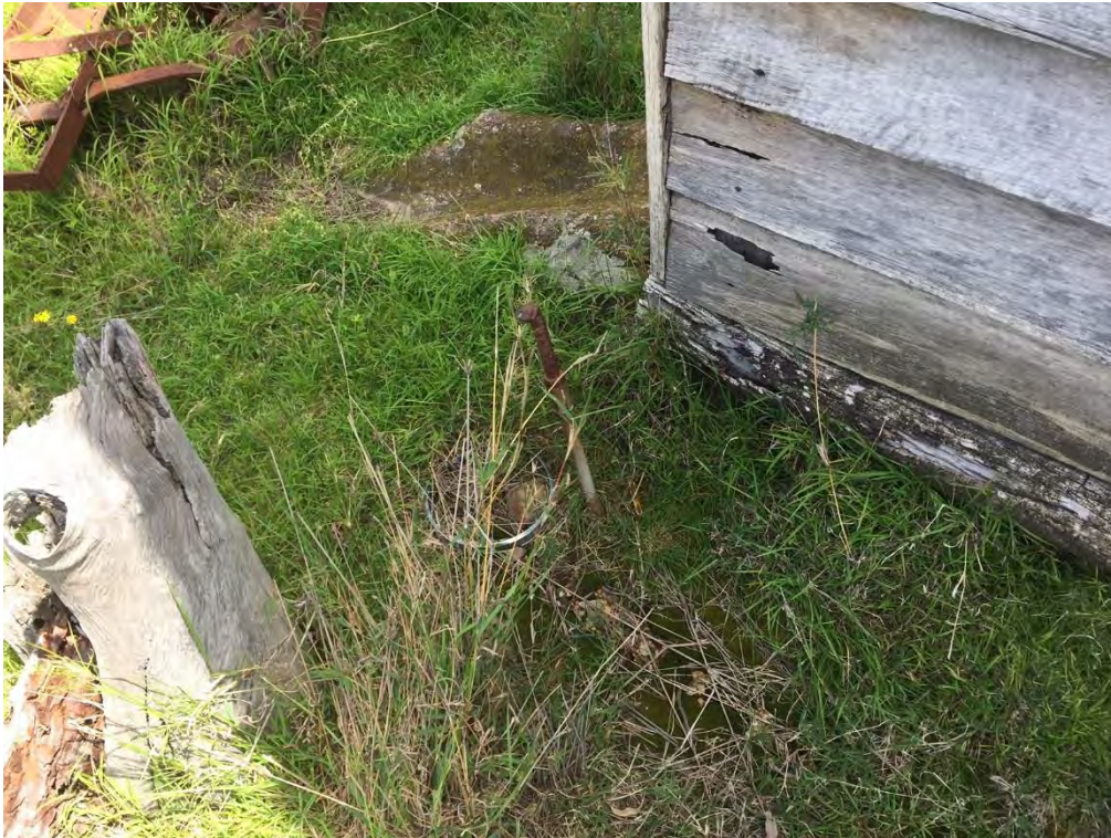
Photograph 15 – Concrete drain from inside of shed and metal stake (unknown purpose)
