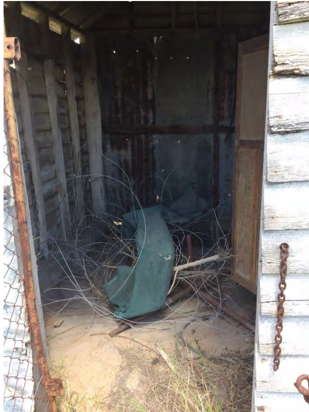
Photograph 13 – Interior of slaughter shed with cupboard, scrap metal and fencing wire and shade cloth
