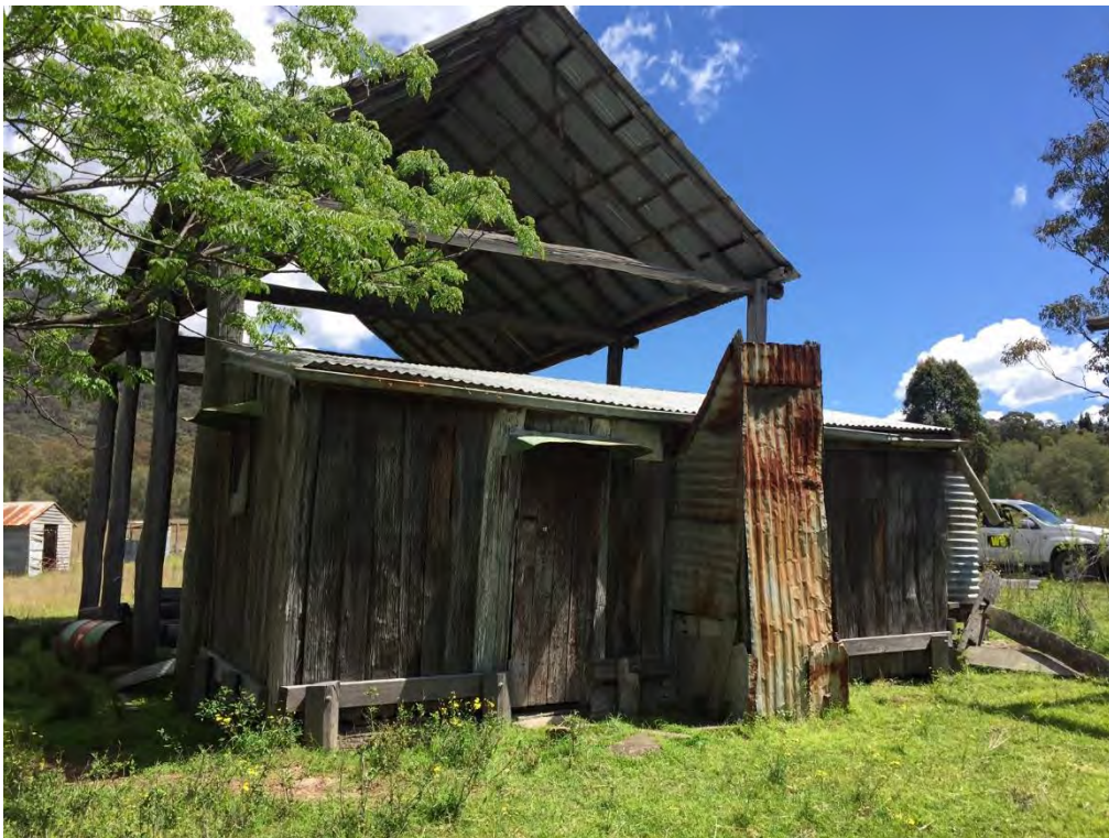
Photograph 2 – Timber shed with rear annexe, fire place and water tank. Empty drum visible on left hand side.
