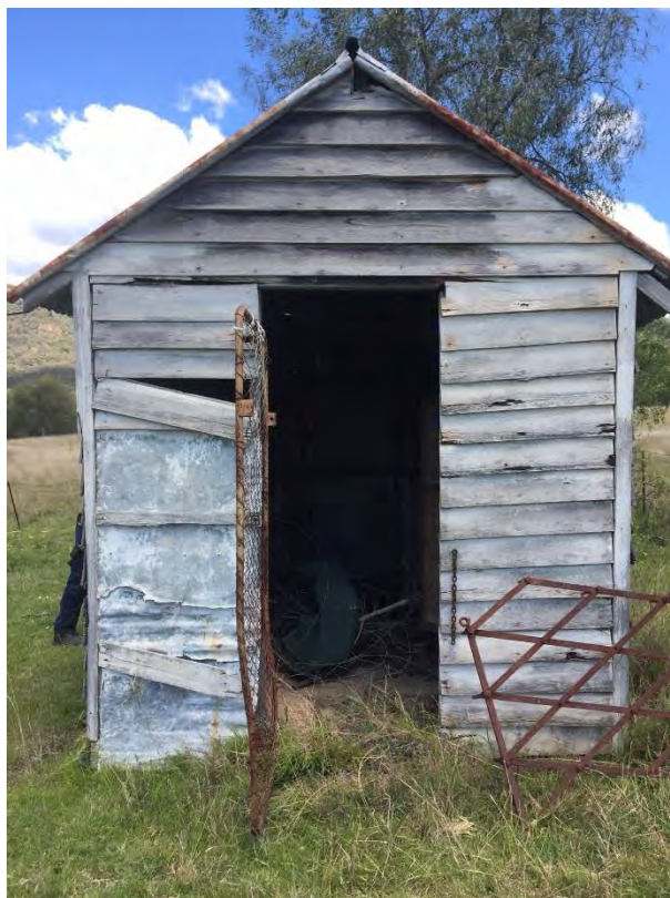
Photograph 12 – Small shed with concrete slab and rear drain. Potential tool or equipment shed or slaughter shed.
