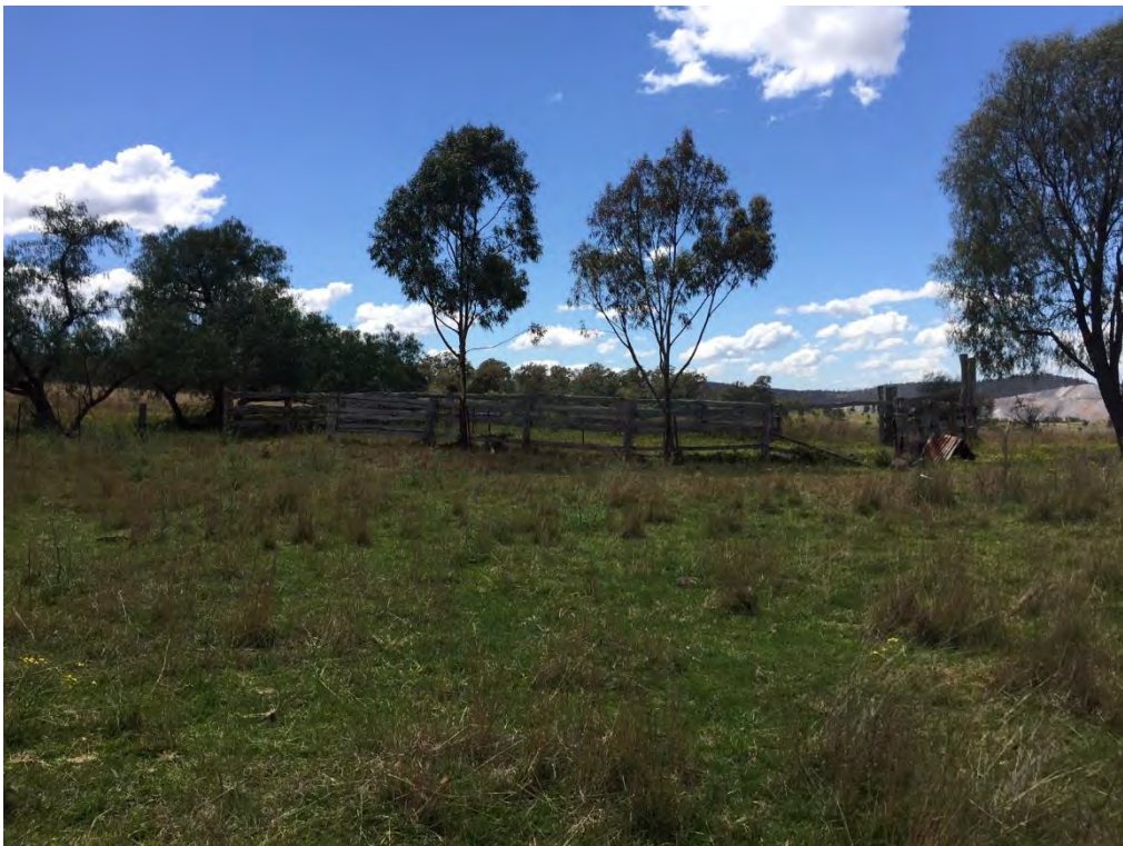
Photograph 10 – Timber stockyards to the far north of the timber shed.
