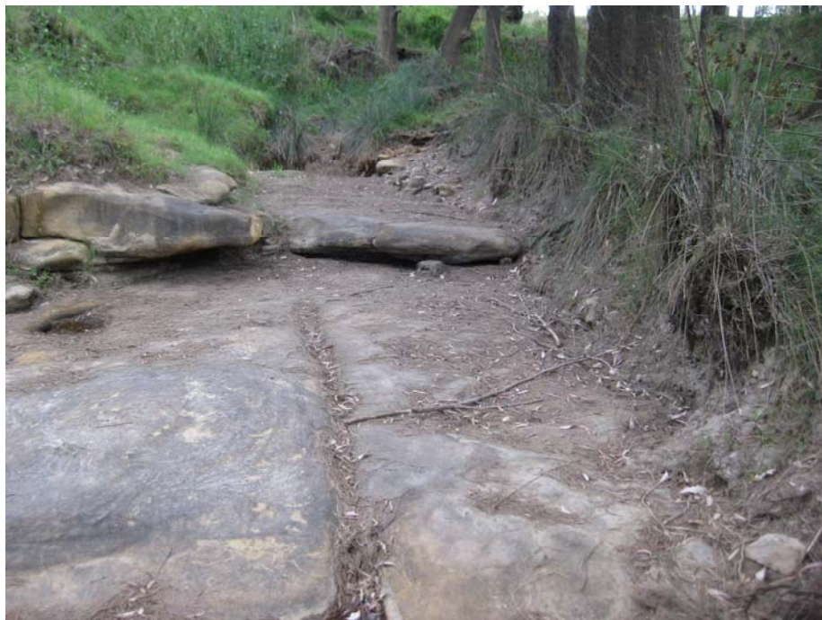
Plate 15: Rock bar in North Wambo Creek (S32°35'31.15" E150°59'48.49", looking upstream)
