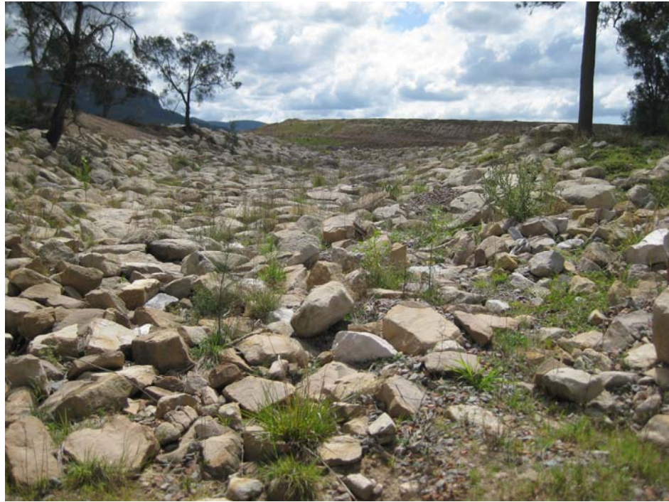
Plate 2: Discharge zone from North Wambo Creek Stage 3 Diversion (looking upstream)
