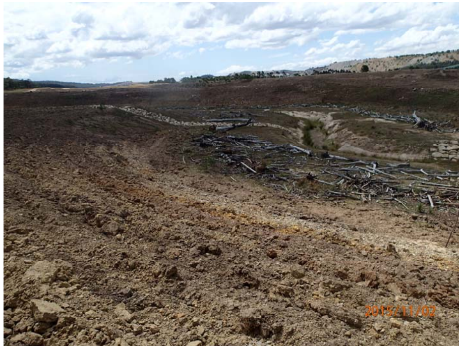
Plate 1: Downstream end of North Wambo Creek Stage 3 Diversion (looking upstream)
