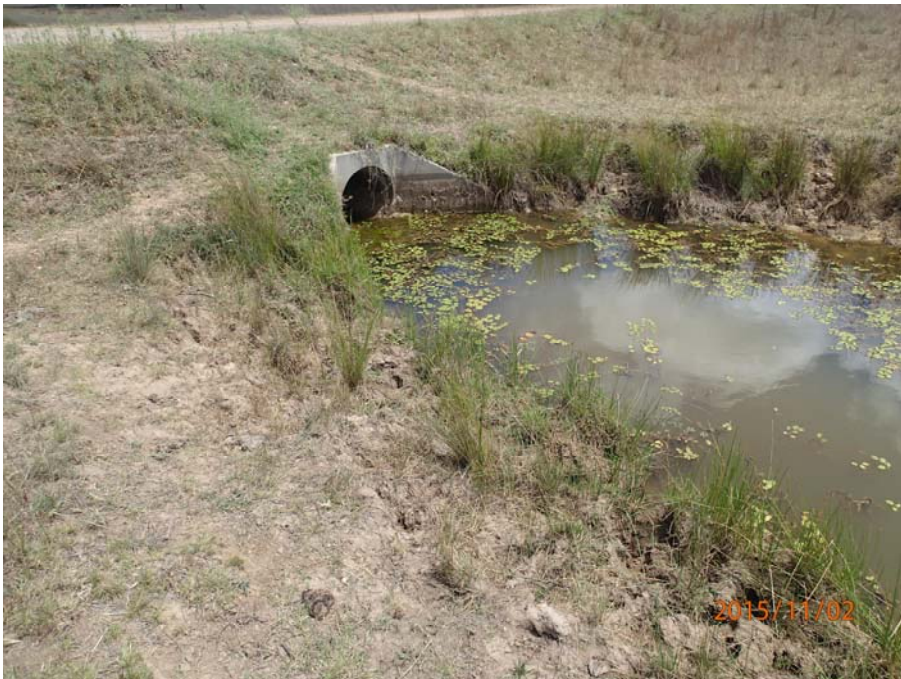
Plate 61: UW1 Culvert crossing of Wambo Road, downstream side
