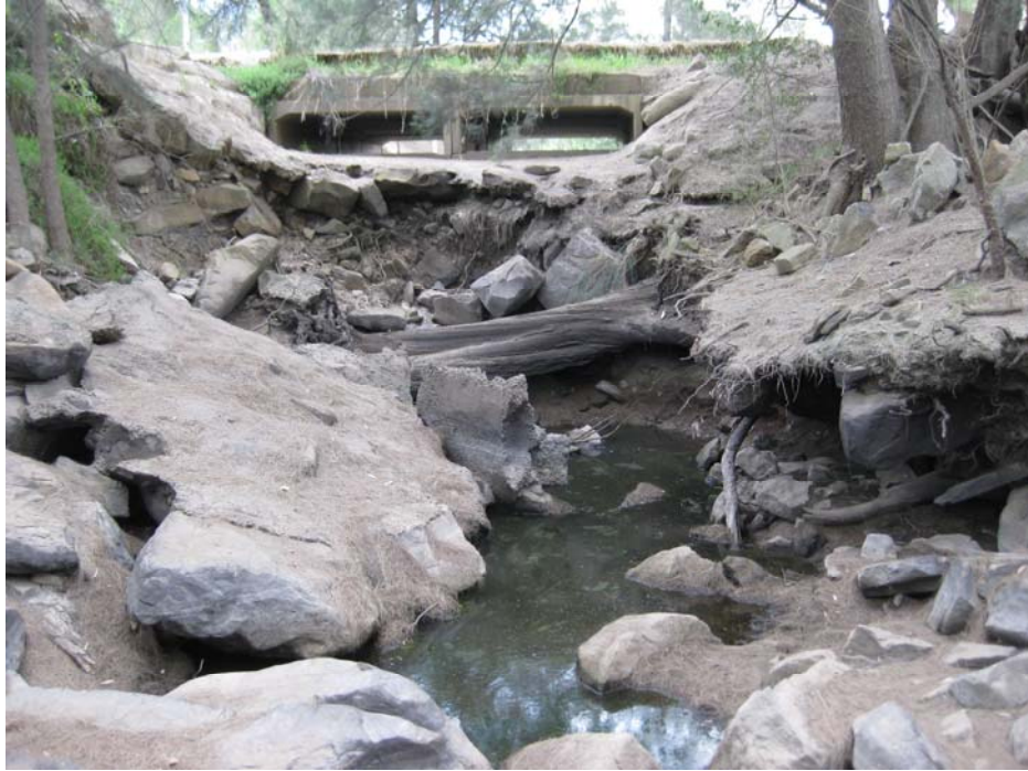
Plate 14: Road Crossing on North Wambo Creek (looking upstream)
