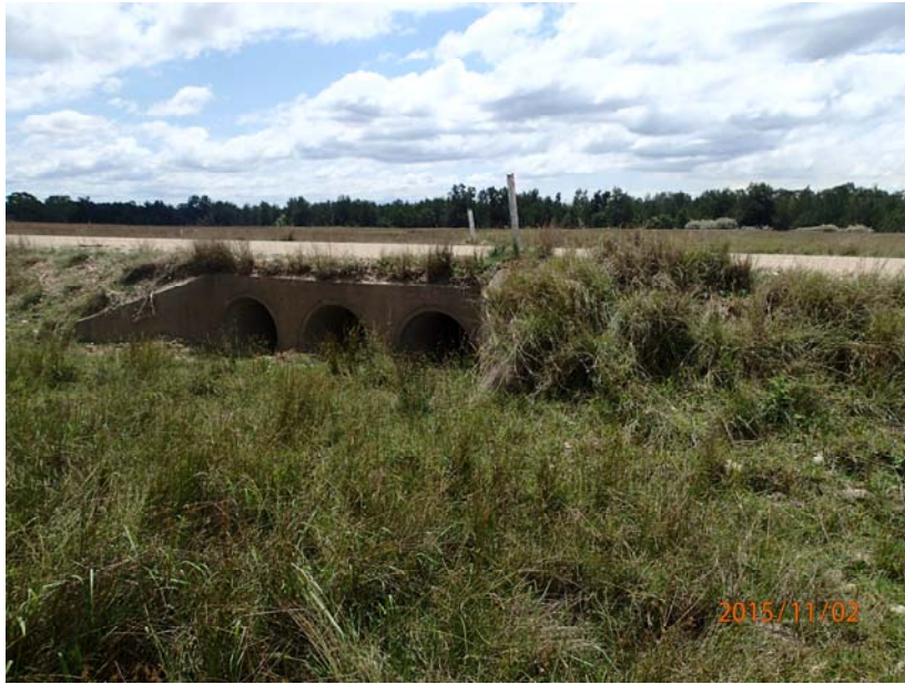
Plate 69: UW3 – Culvert under Wambo Road
