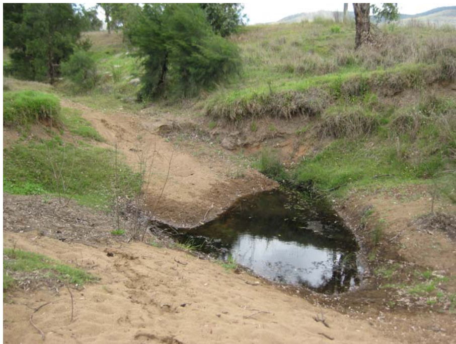
Plate 52: Wambo Creek – permanent pool and eroded banks upstream of Wambo Road (looking upstream)
