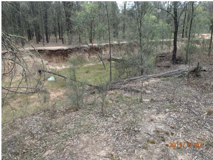
Plate 5: Small unnamed tributary of North Wambo Creek, with degraded channel and erosion (looking downstream)
