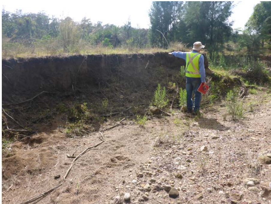
Plate 27: Eroded vertical banks to main channel in Stony Creek (looking downstream)
