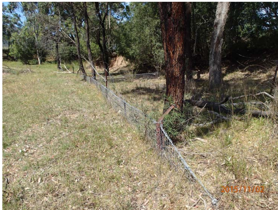
Plate 36: Bank stabilisation works in Stony Creek (S32°36'10.81" E150°58'13.73", looking downstream)
