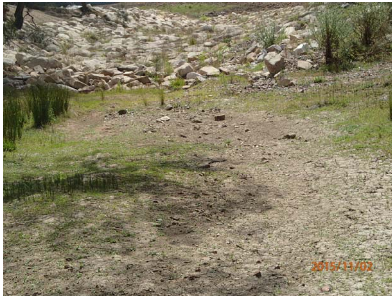
Plate 3: North Wambo Creek channel below Diversion (looking upstream)
