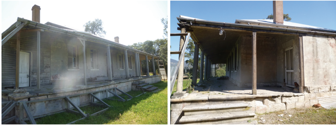
Fig. 6.8 Homestead Building Structure
