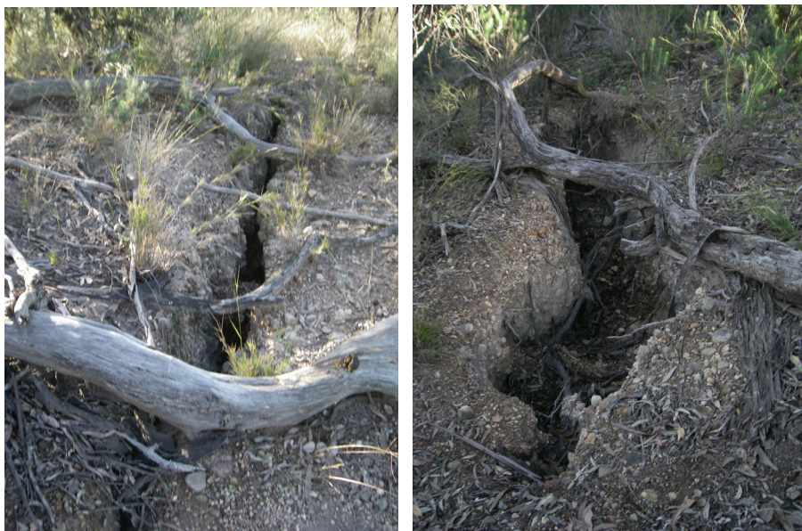
Fig. 4.6 Photographs of Surface Cracking at the NWUM
