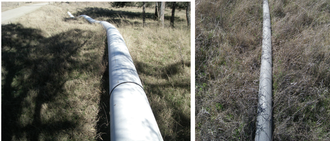
Fig. 6.2 Photographs of the Water Pipelines
