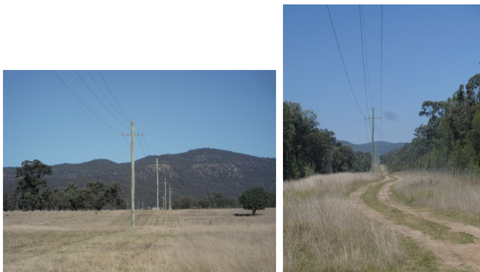
Fig. 6.3 Photographs of the 11 kV Powerlines
