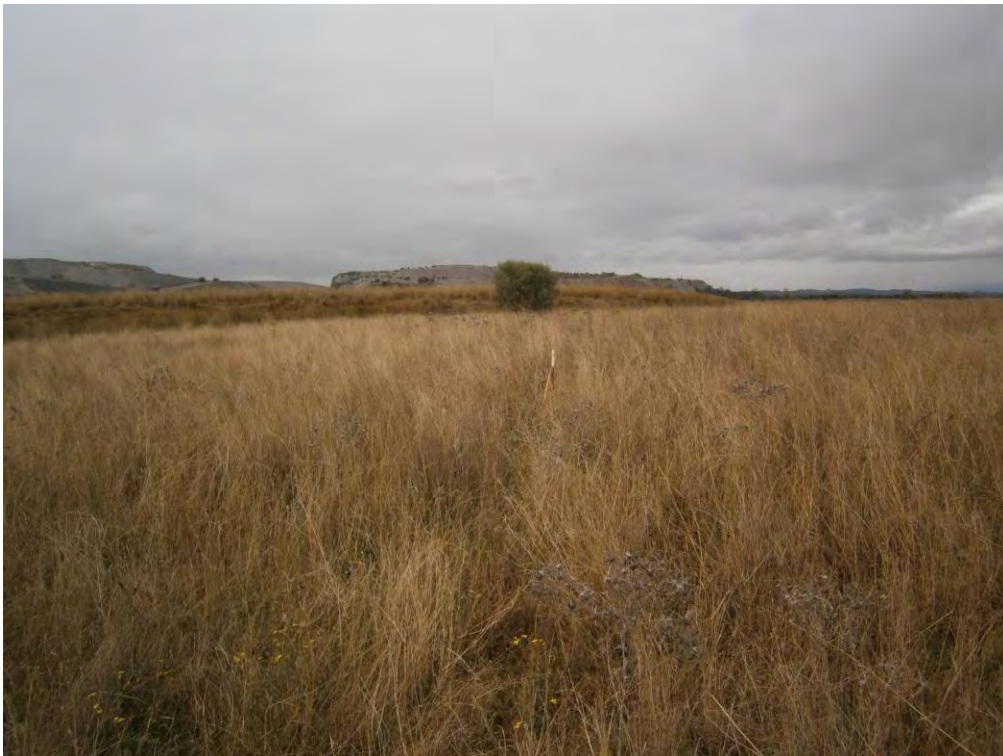
Plate 10: Survey Unit 2 - View north east showing modified contour bank and North Wambo Creek Diversion works.
