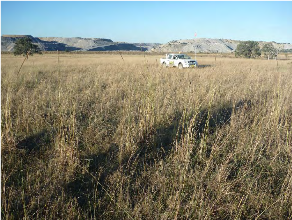
Plate 3: Survey Unit 1 - View north east showing modified contour bank and North Wambo Creek Diversion works near the open cut mine area.
