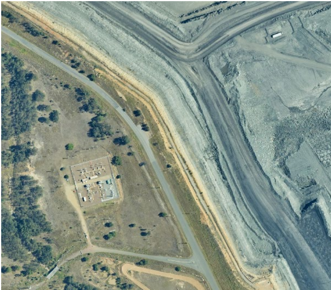
Figure 3-1 – Newdell Zone Substation proximity to mining operations 9Aerial Photo date Jan 2018Planning
