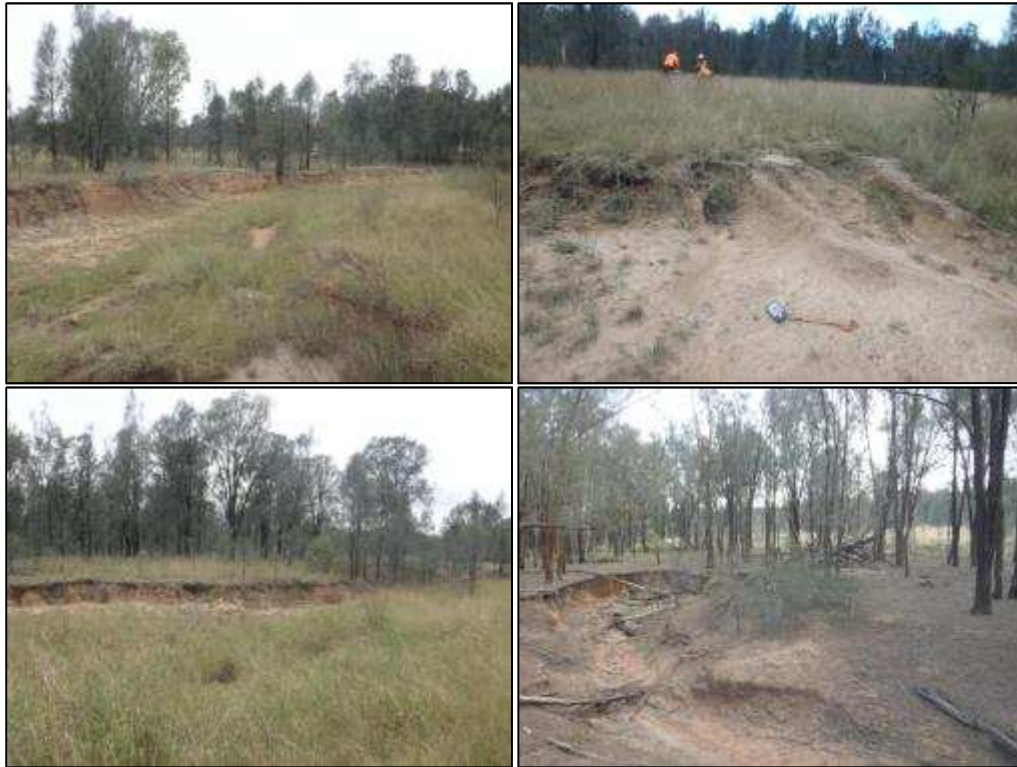
Plate 1: LID 3: Erosion gully where surface manifestation of site was identified.
