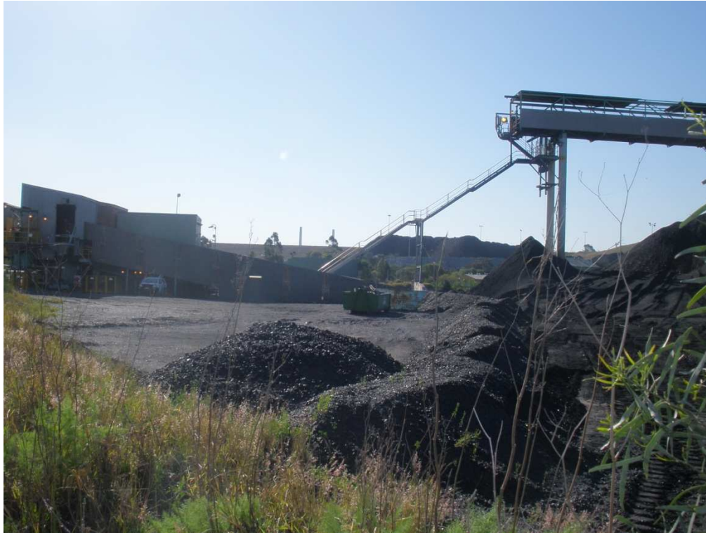
Plate 25: CHPP Pit area.
