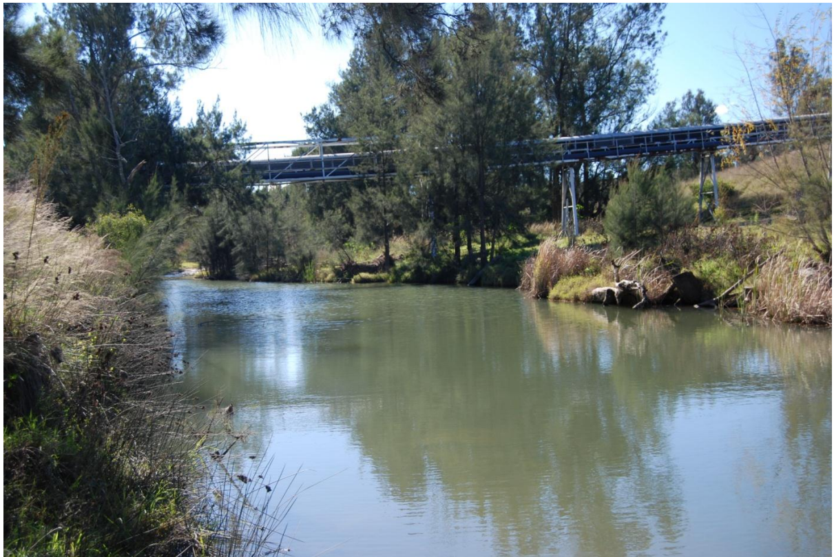
Figure 19. Bowmans Creek at BCK5, looking upstream.
