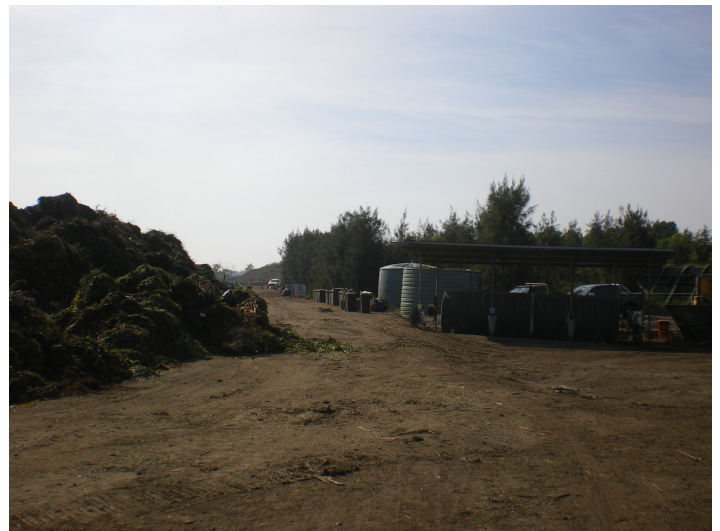
Photo 2: Refuelling facility and water tanks (Source: WSN)
