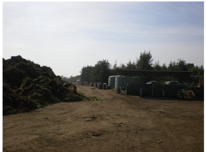
Photo 2: Refuelling facility and water tanks (Source: WSN)
