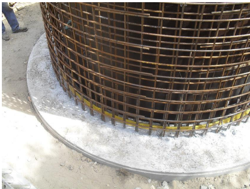
Steel formwork of lift/cutting ring tied in to lower ring
