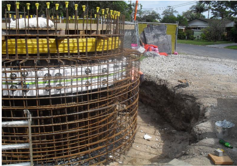
Steel formwork of lift/cutting ring before concrete pour
