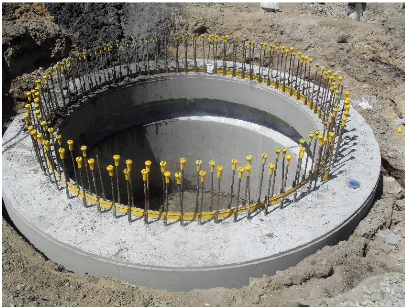
Lift/Cutting ring post excavation to sink ring
