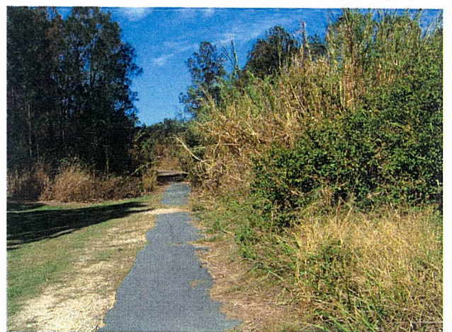
Plate 6: pipeline route near sewage treatment plant
