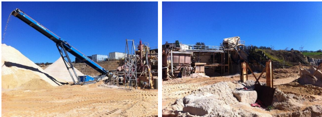
Figure 2-1 Existing Processing Plant
