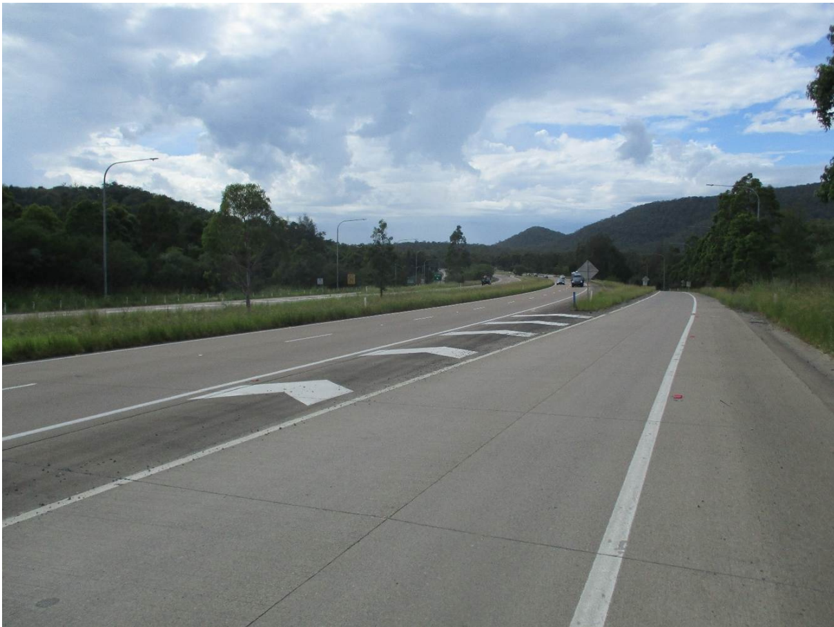
Photograph 3: A1 Pacific Highway near Tarean Road north interchange, Karuah.
