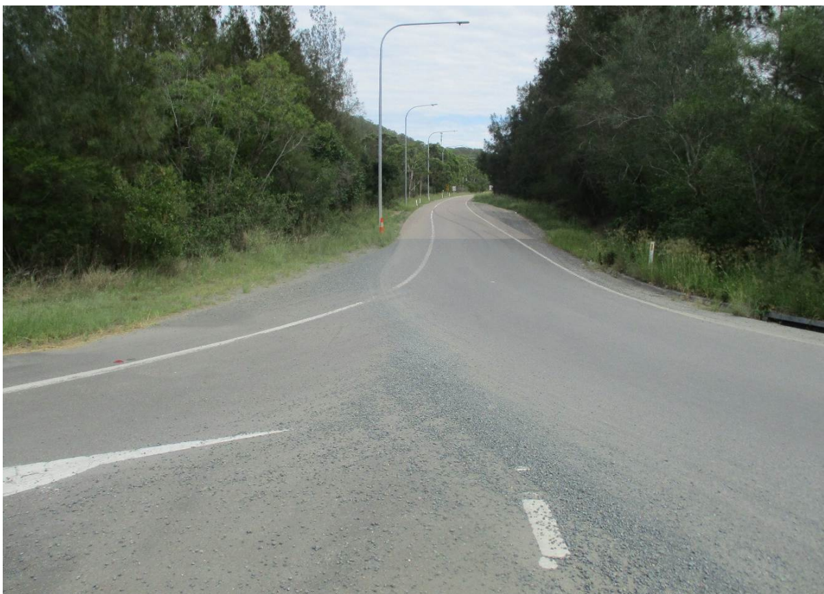
Photograph 4 – A1 Pacific Highway - Tarean Road north southbound on-ramp.
