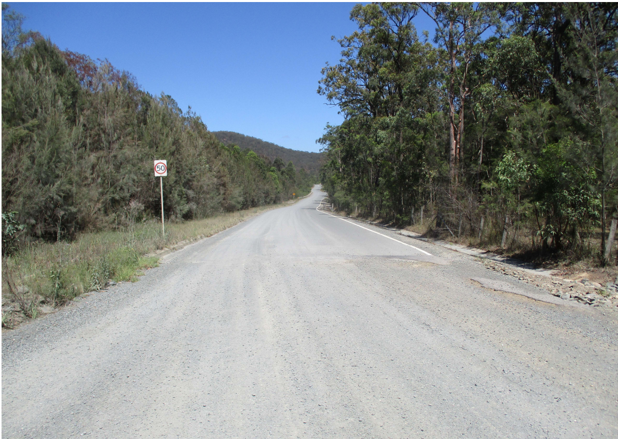
Photograph 8 – Blue Rock Close near Karuah East Quarry entrance.
