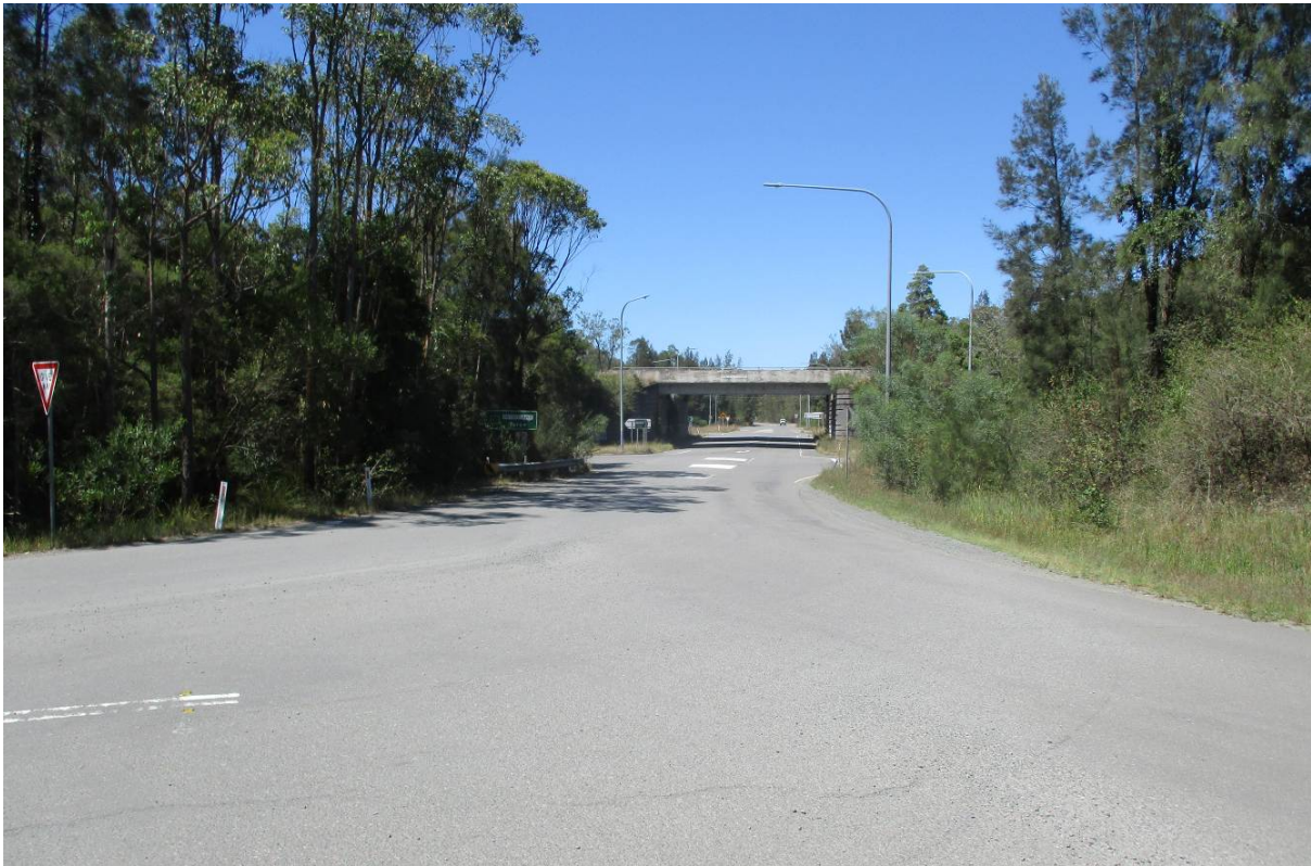
Photograph 6 - Tarean Road north near A1 Pacific Highway interchange.
