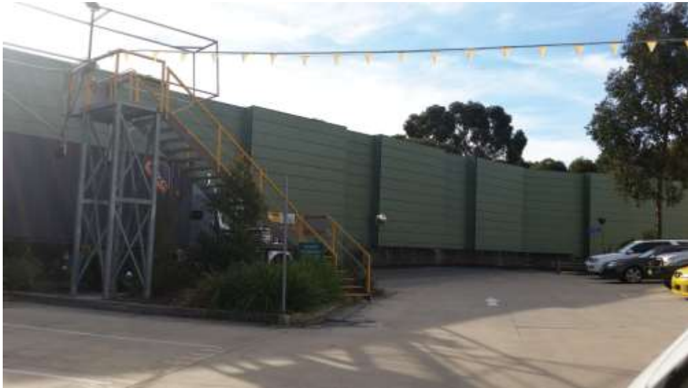
Figure 11 Existing acoustic fence to rear (west) of Building 8B
