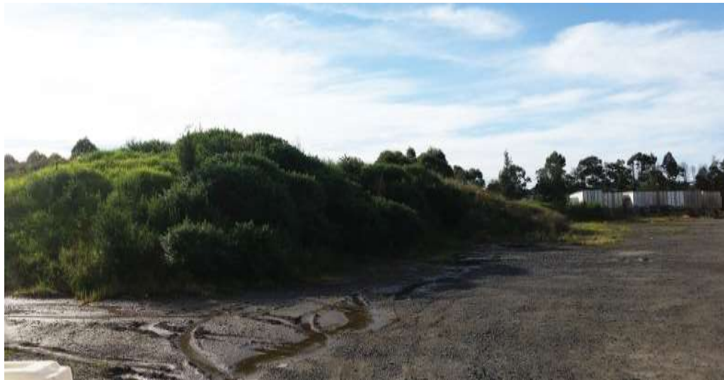
Figure 9 Existing mound to be removed to make way for proposed Building 8A
