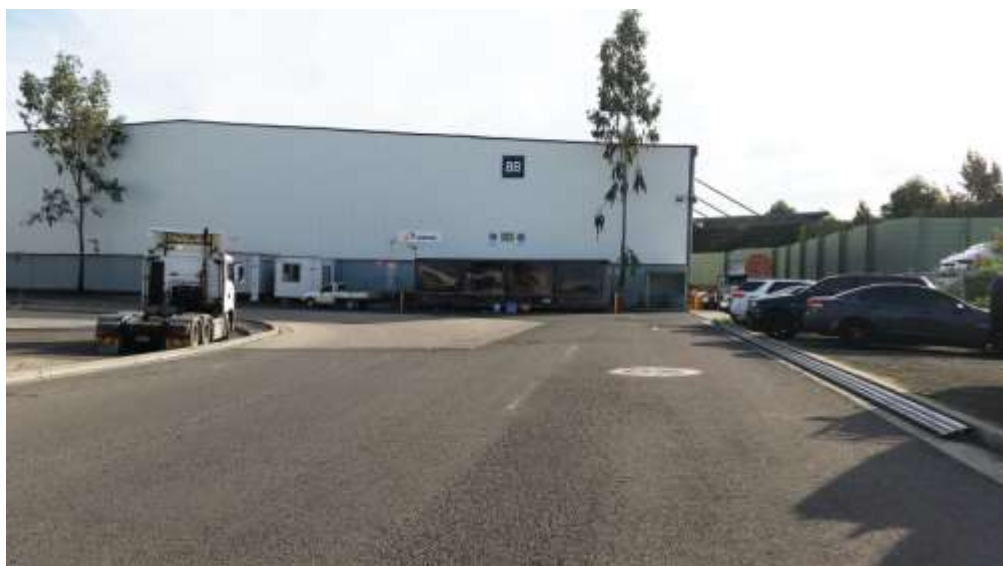
Figure 10 Looking west towards Building 8B and existing acoustic fence
