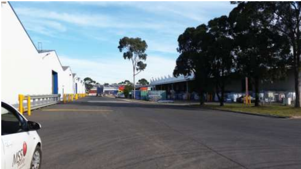
Figure 12 Looking south along access way between Buildings 2 and 3
