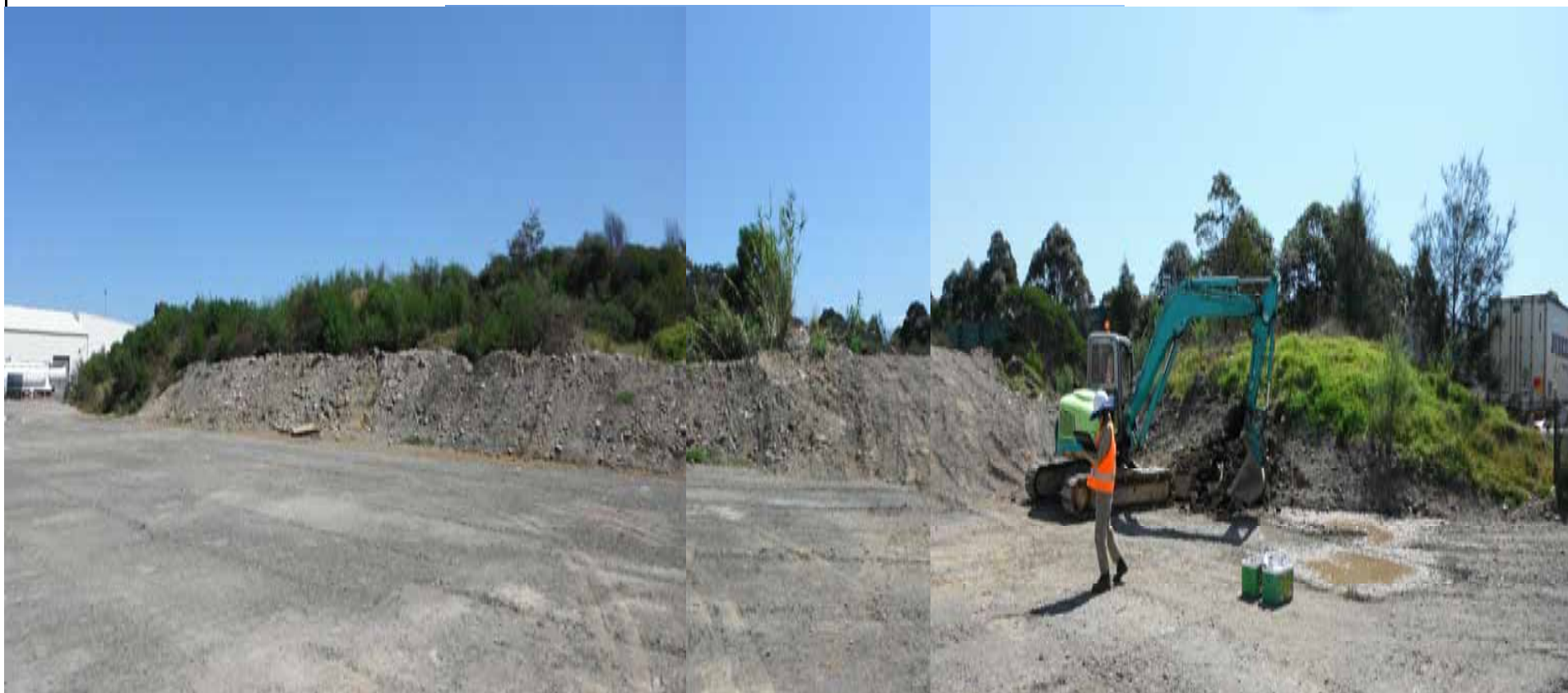
Panoramic view of the existing earthen mound located in the north-western portion of Yennora Distribution Centre site
