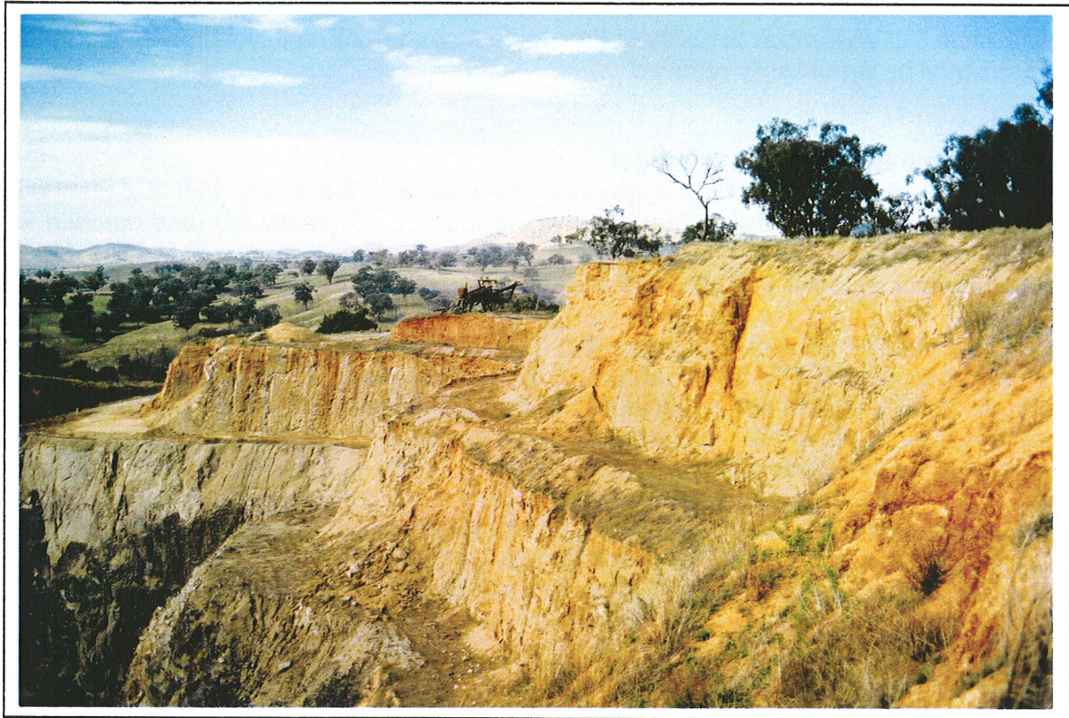
Plate 3.2 Current stormwater diversion around the top benches of the void (Ref: 509B/15)
