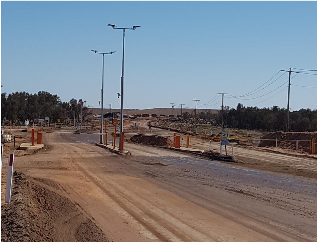
Figure 28 – Ginkgo/Crayfish Mine main entrance security boom gates
