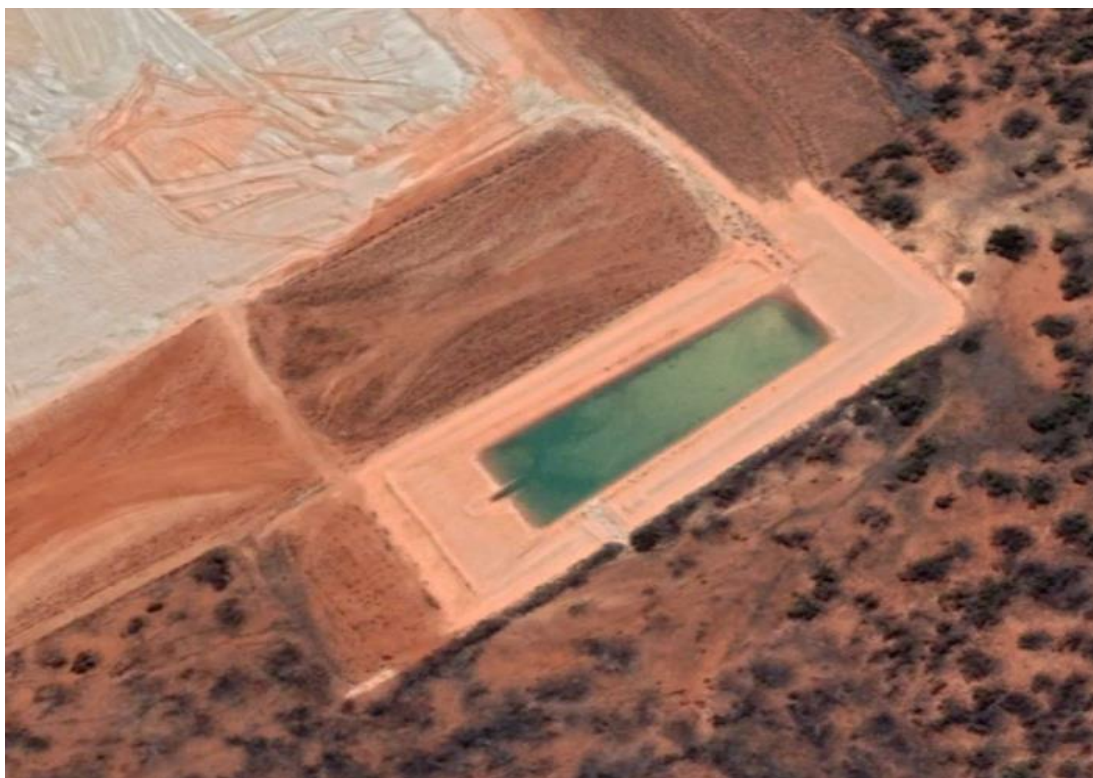
Figure 11 – Sediment Pond at Crayfish Mine
