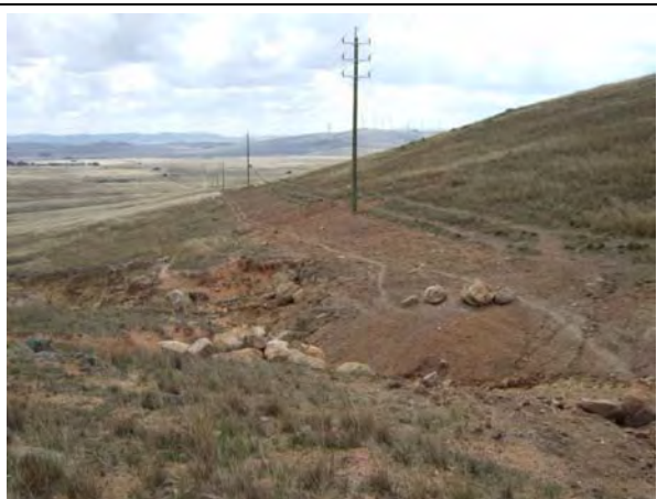
Plate 6.7 – Double circuit 33 kV overhead line from Ellenden to Grose Hill. Visibility of the line reduces with distance.
