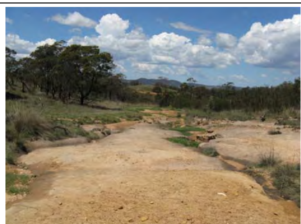
Plate 5.14 – Existing track erosion near Turbine 1
