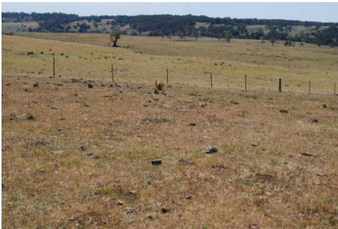
Photograph 2. View along cable route northeast from substation site to power line start.
