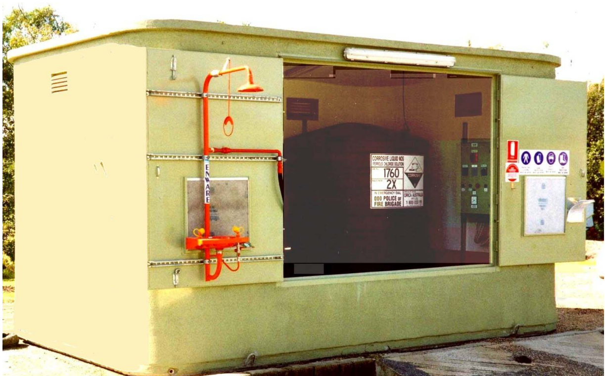
Figure 2.2 – Example of a Typical Chemical Dosing Facility
