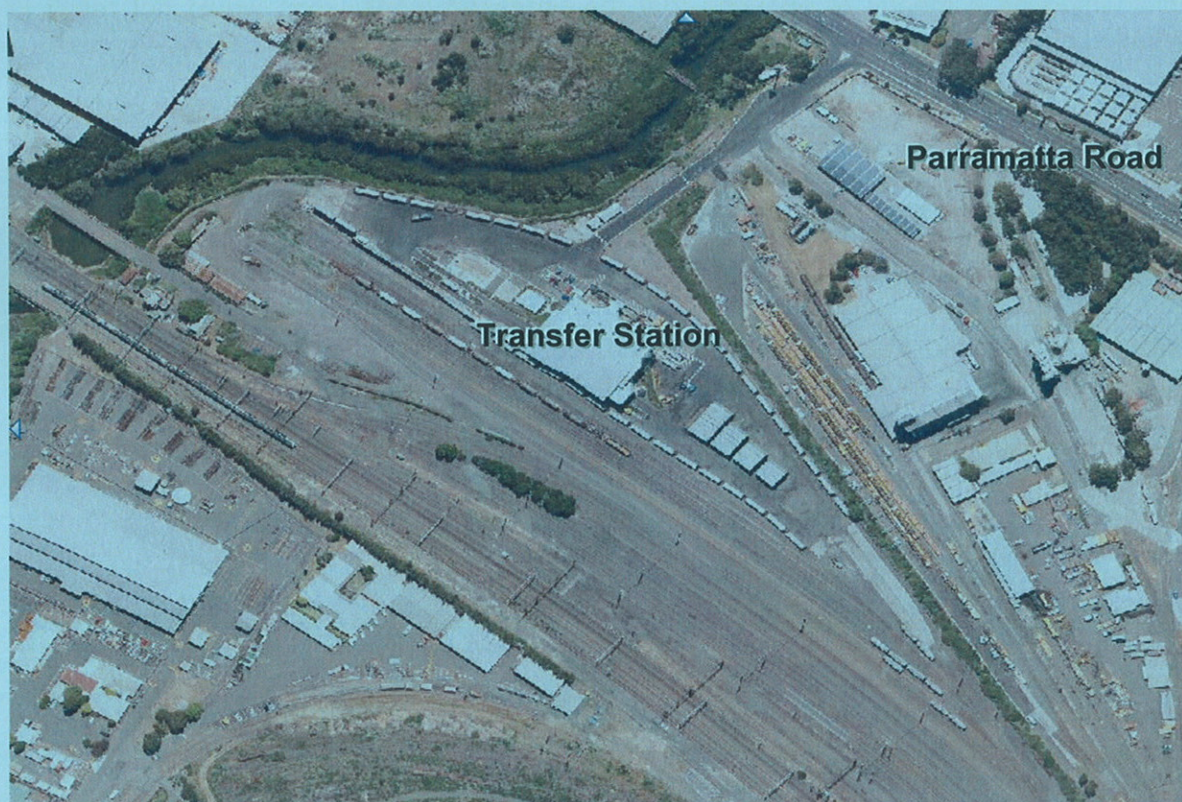
Figure 1 - Clyde Waste Transfer Station
