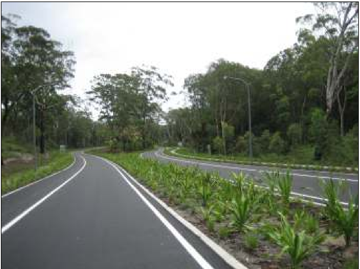
Existing access road (facing Nelson Bay Road) with ecological corridor on right.
