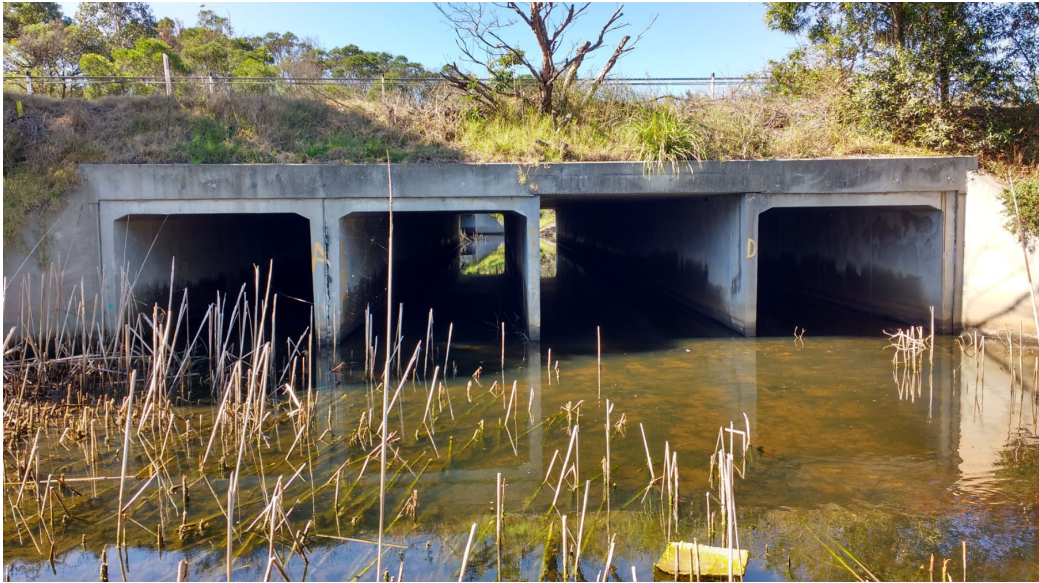
Figure 4.4 Culverts beneath Princes Highway
