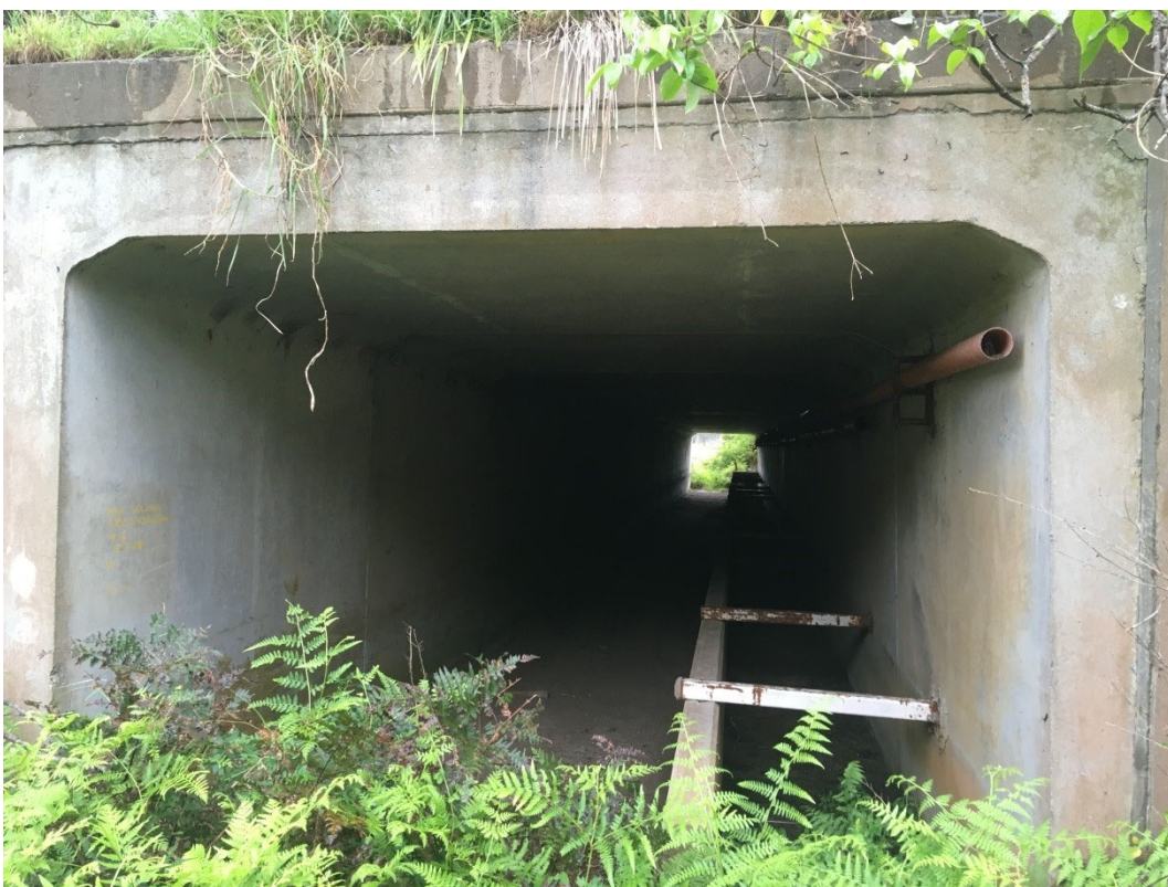
Figure 4.5 Swamp Road culvert
