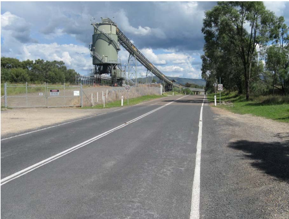
Plate 2. Watt Street looking toward Wambo Coal mine, and showing train loading facility to the left.
