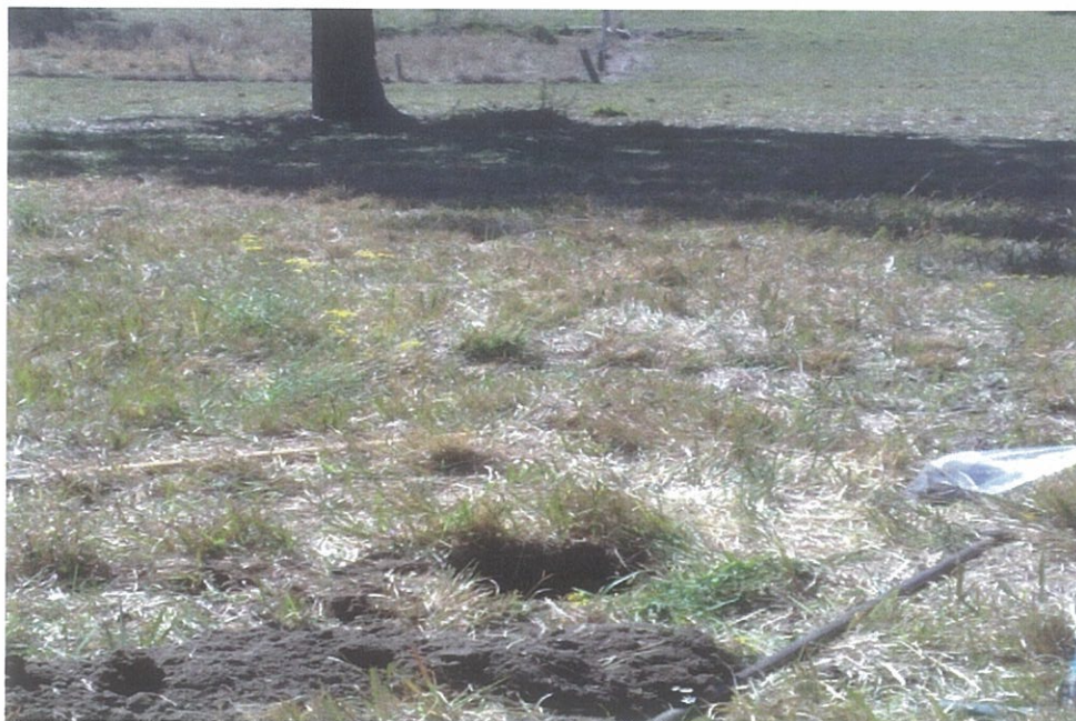
Bore Hole 1 First Sample View: North West
