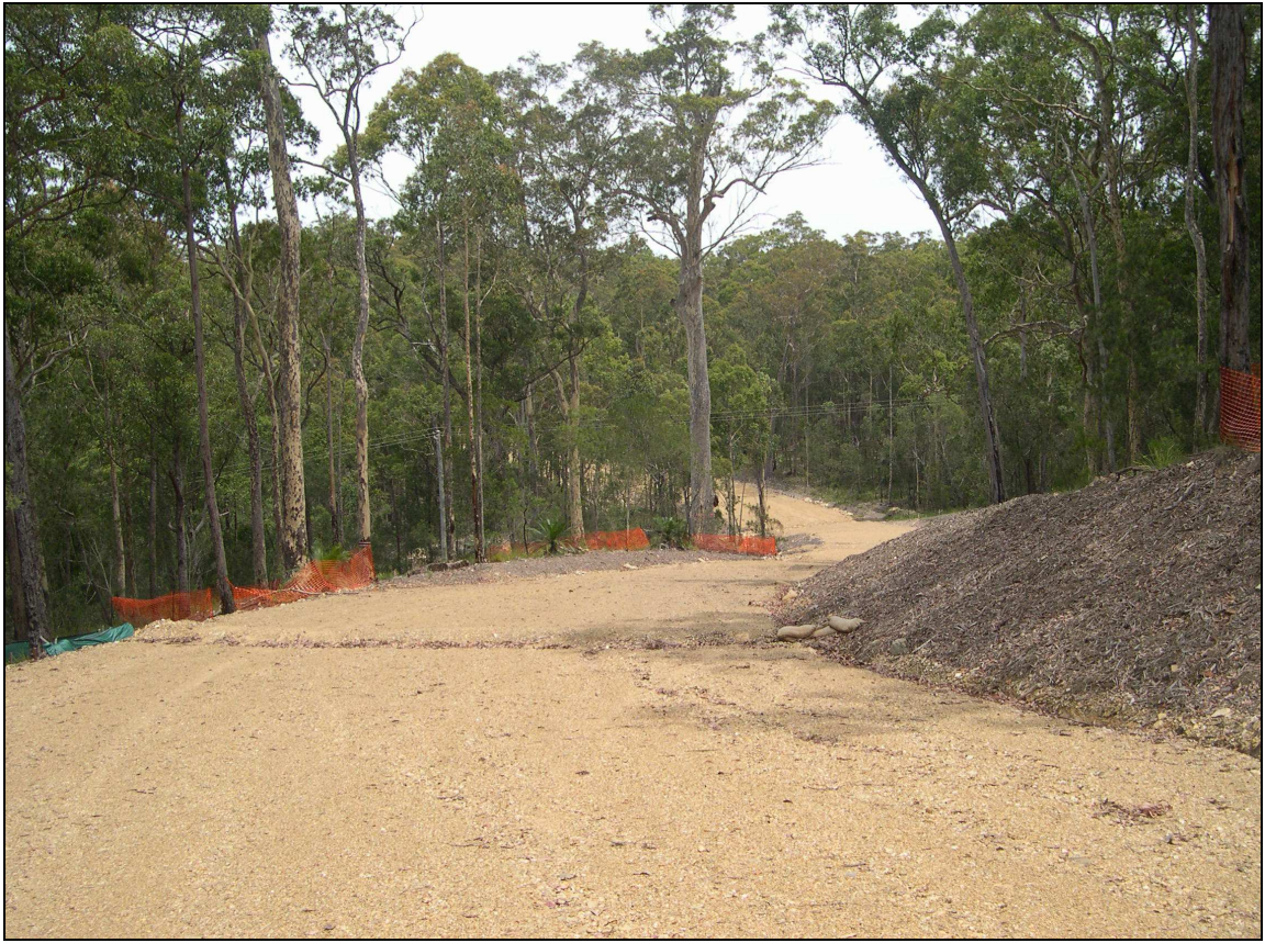
Figure 4: The Site – existing internal road under construction
