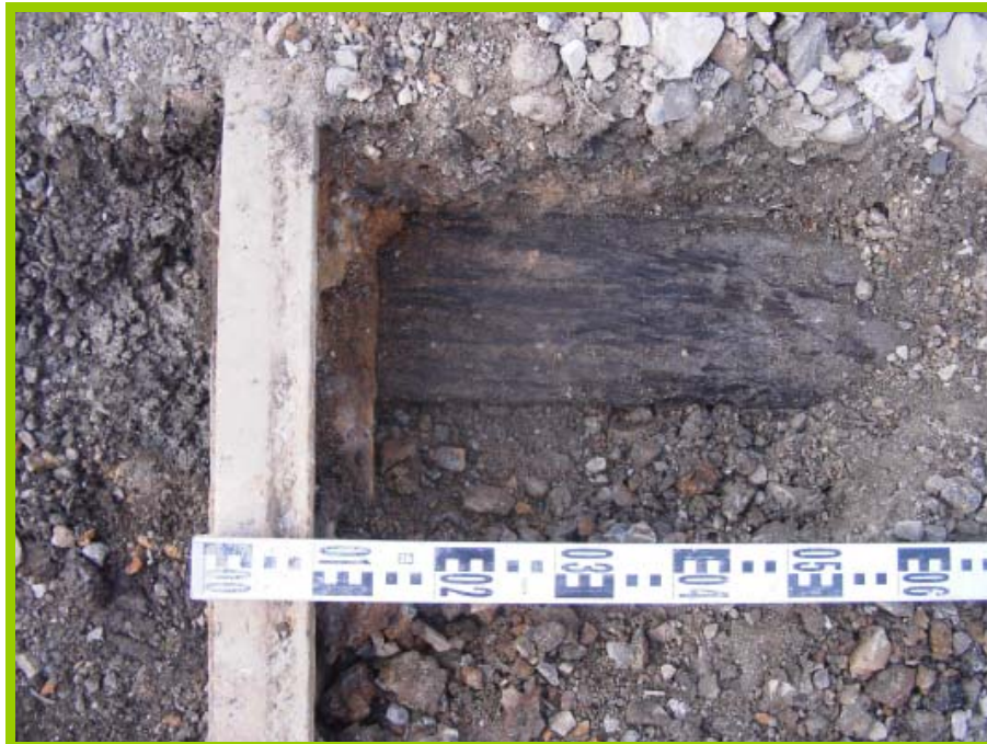
Figure 12: Tram rail and partial sleeper 23
