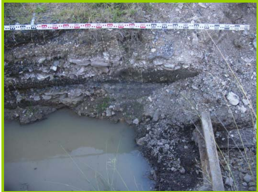
Figure 11: Tram rail and partial sleepers on right with layers of later asphalt and fill 22
