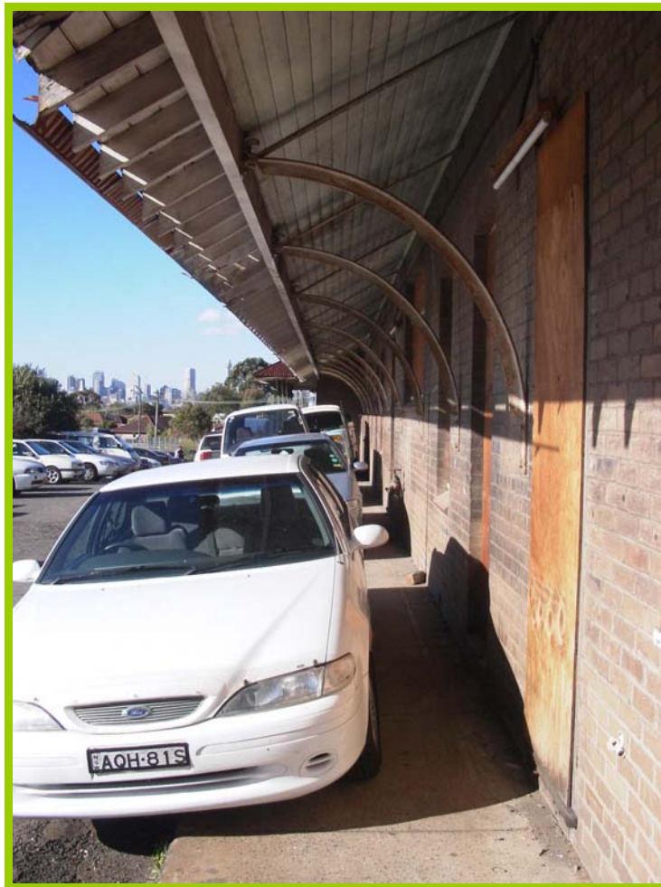
Figure 10: Verandah of Traffic Office with iron supporting brackets 17
