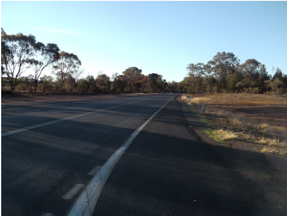
Photograph A.58 West Wyalong Condoblin Road/Ungarie Road/Wamboyne Road intersection – looking north towards West Wyalong Condoblin Road
