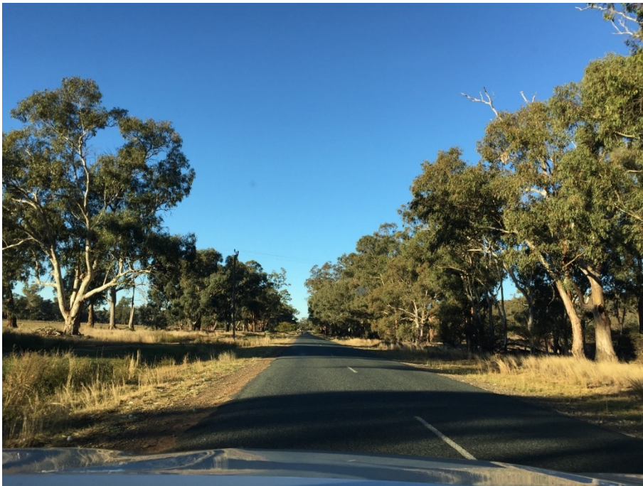
Photograph A.53 Lachlan Valley Way, sealed road with only centre line marked
