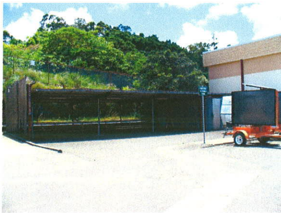
Figure 3-2 Car Park on the western side of the Building
