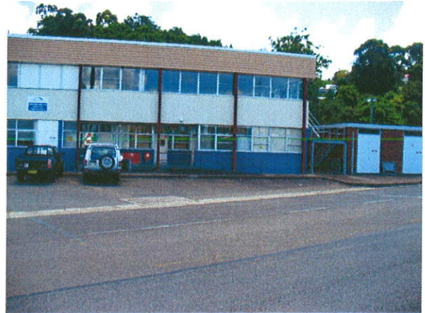
Figure 3-3 Eastern end of the Building with adjacent electrical supply room
