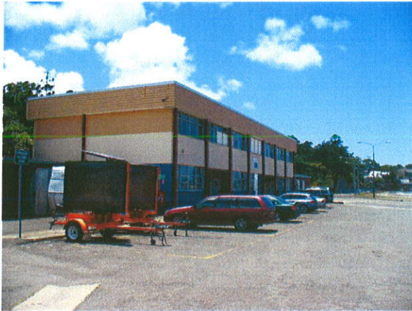
Figure 3-2 Office and Amenities Building facing north
