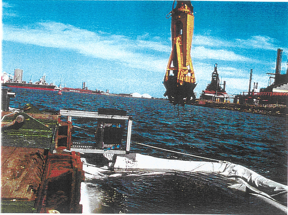
Photo 1 Dredging simulation process
