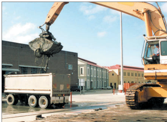
Plate 6.9 Excavator working in conjunction with trucks
