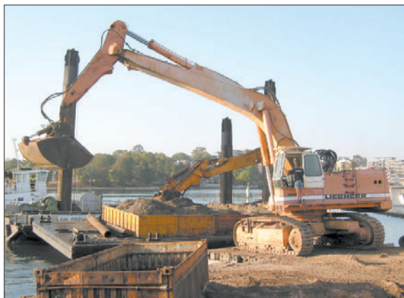
Plate 6.5 Example of dredge in operation - excavator unloading flat topped barges
