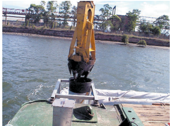
Plate 17.2 Dredging material filling to the container
