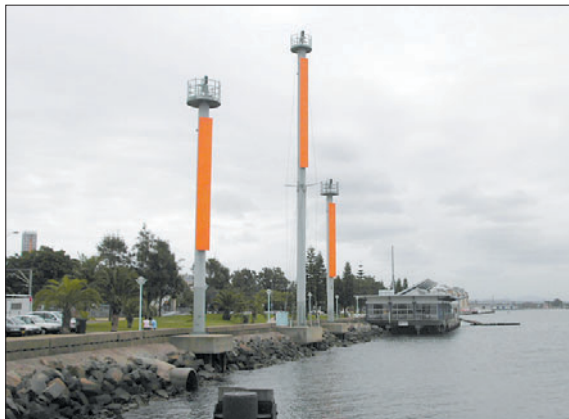
Plate 6.1 Example of navigation aids - main channel leads
