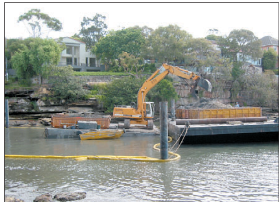
Plate 6.4 Example of dredge in operation - excavator on a barge
