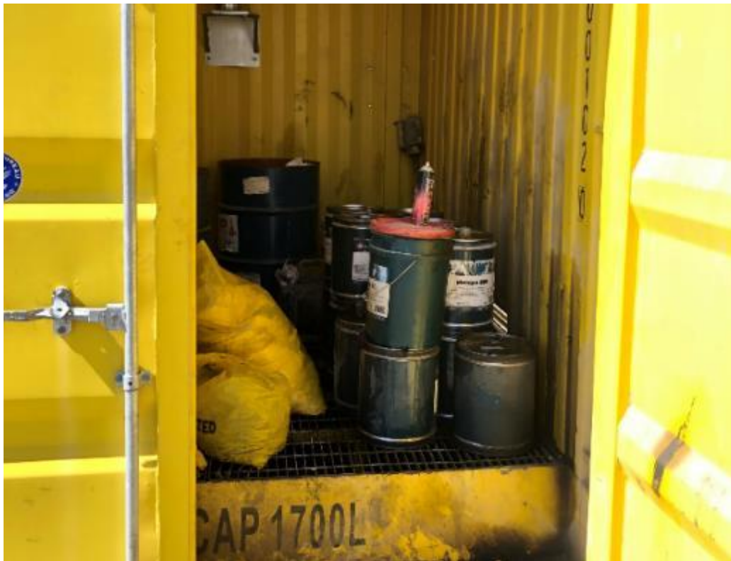
Figure 14: Storage of oils within bunded containers
