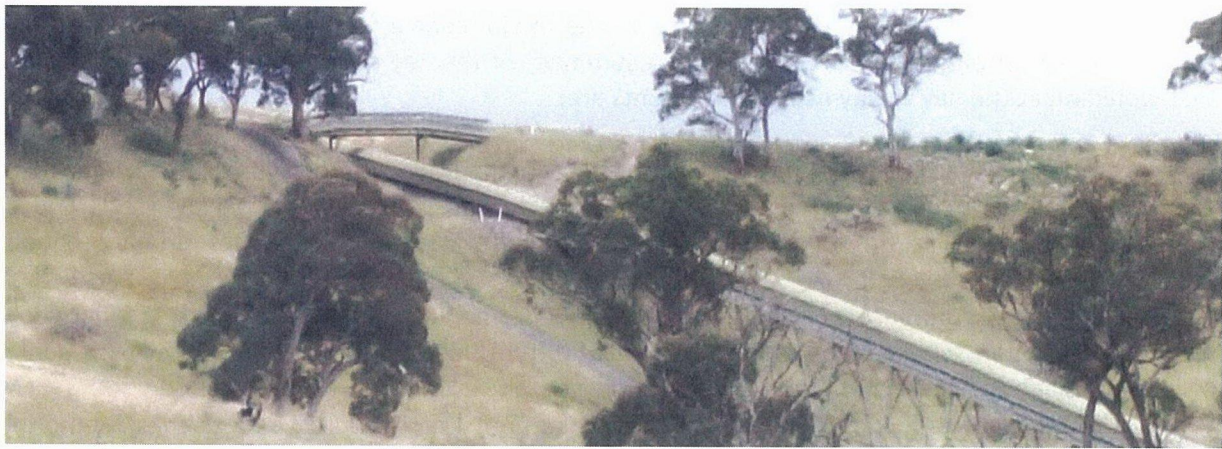
Mine related infrastructure is visible throughout the area.
