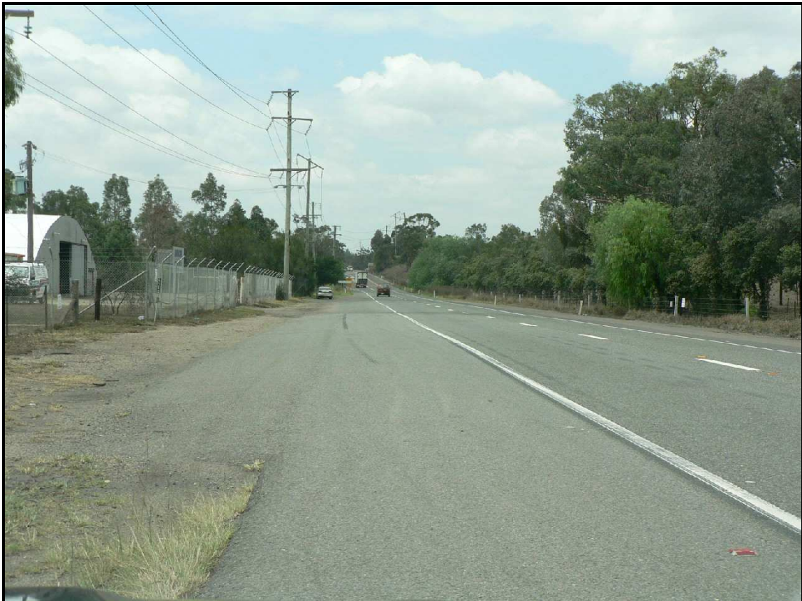
The New England Highway looking south in vicinity of existing access locations (Note wide sealed road shoulders)
