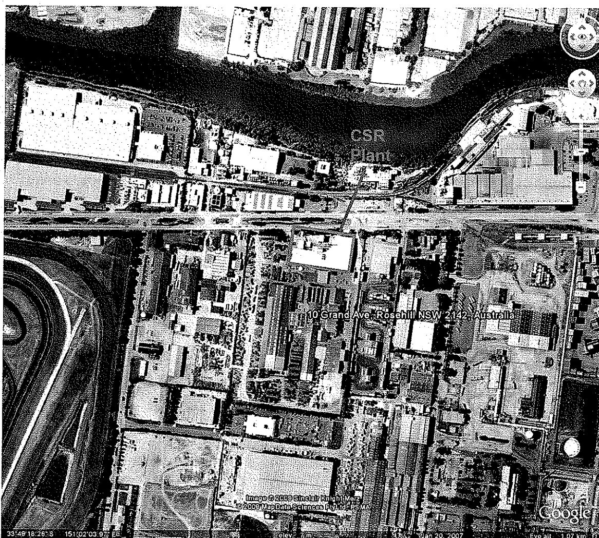
Figure 1 – Approved CSR Concrete Tile Manufacturing Plant
