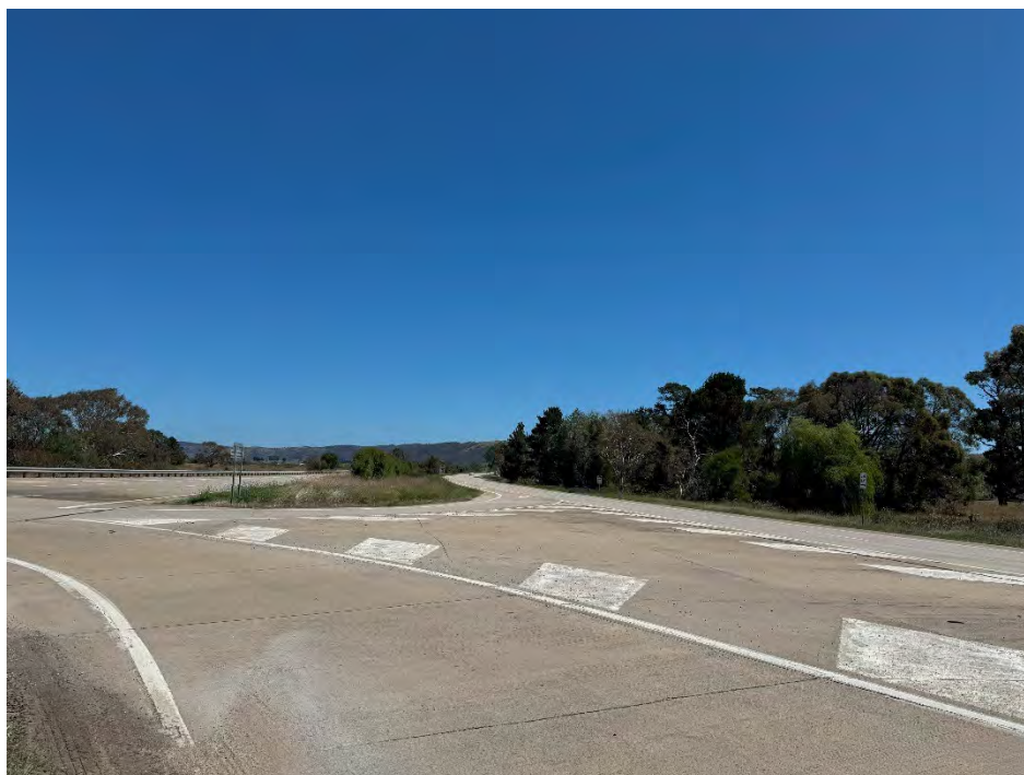
Figure 6 Site Access Monaro Highway looking North
