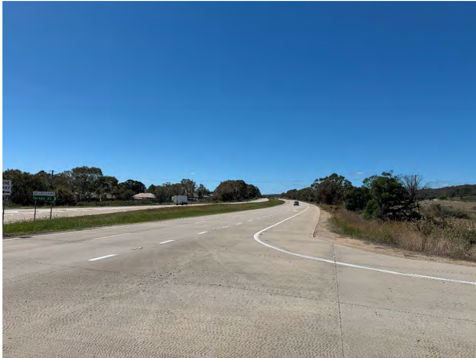
Figure 5 Site Access Monaro Highway looking North
