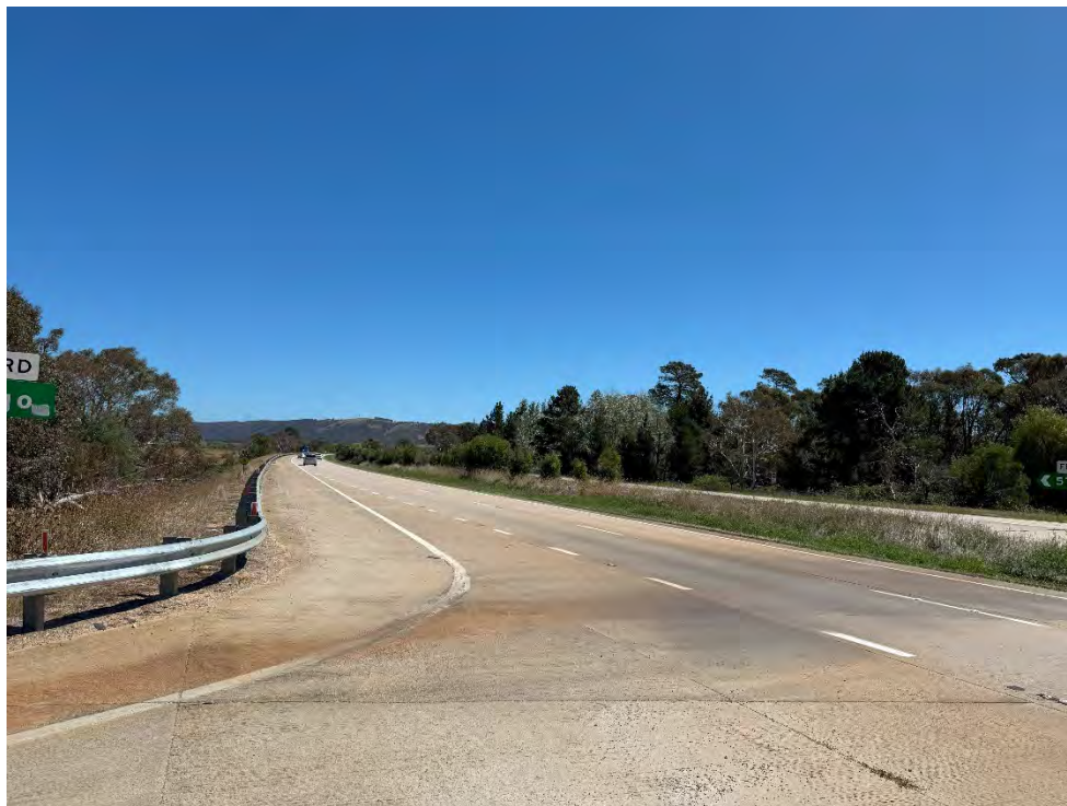
Figure 4 Site Access Monaro Highway looking North
