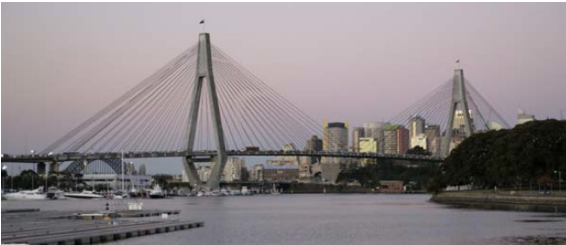
Figure 11: ANZAC Bridge, as viewed from Rozelle Bay, which is to the south-west of Glebe Island (Source: RTA website)
