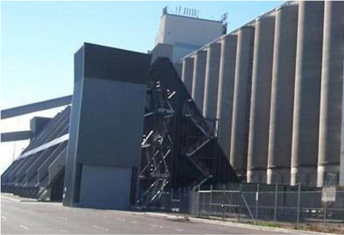
Figure 14: Western side of gypsum handling facility as viewed from Sommerville Road, with the silos to the right of the picture (Source: NSW Heritage Office)
