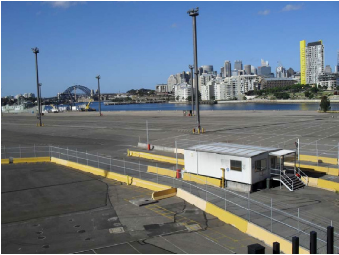
Figure 7: Existing shed at the southern end of the site
