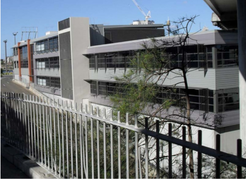
Figure 12: Western side of western wing of the Maritime Maintenance Facility, viewed from Sommerville Road underneath the ANZAC Bridge
