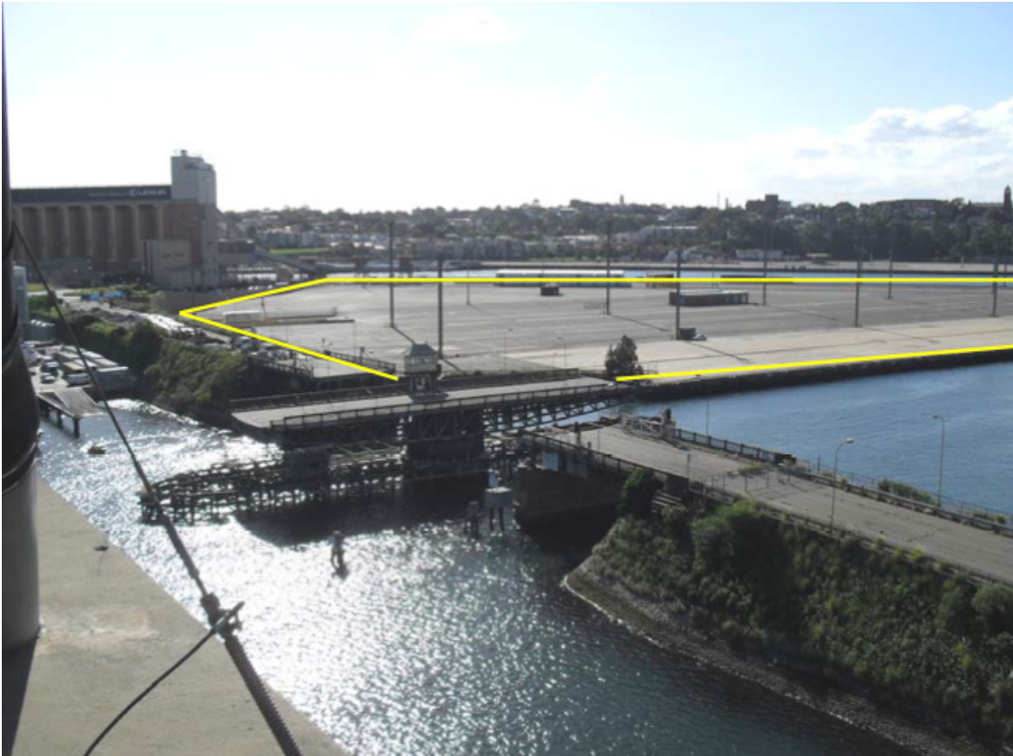
Figure 10: Old Glebe Island Bridge, as viewed from the Anzac Bridge. The subject site is highlighted in yellow.
