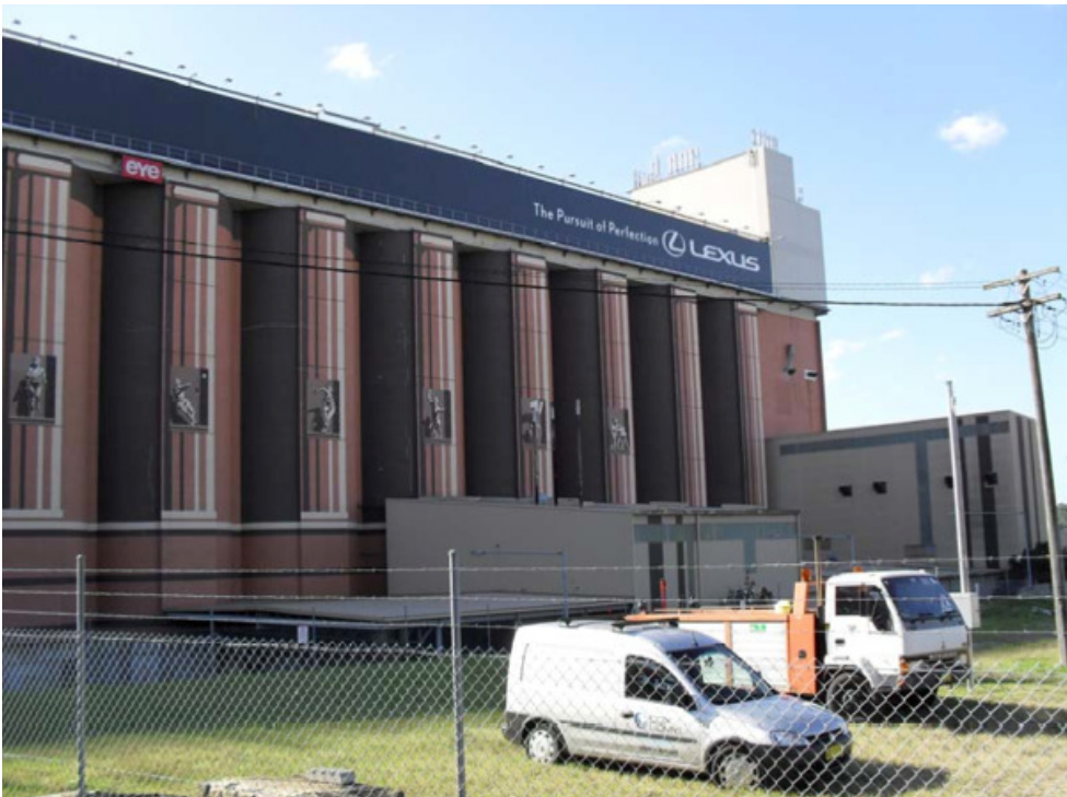
Figure 13: Southern face of former grain silos, as viewed from Sommerville Road
