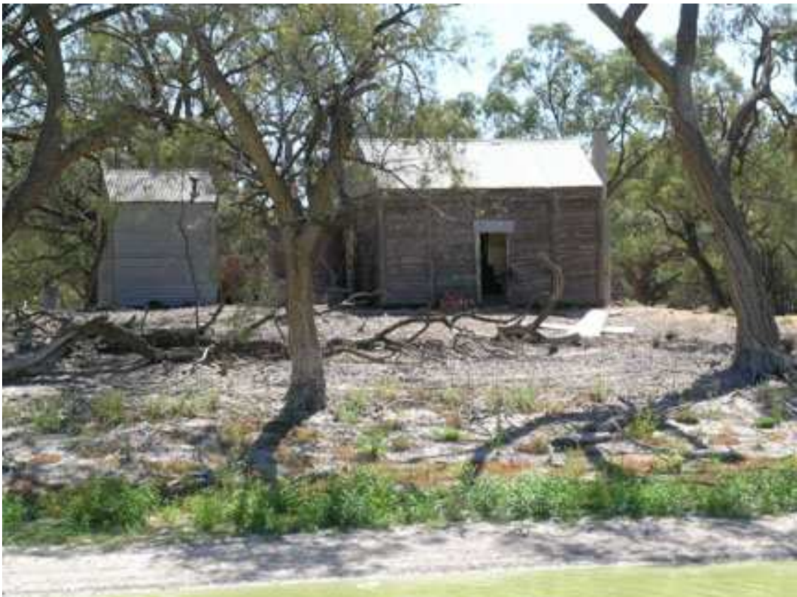
Figure 3. Toora homestead outbuildings.
