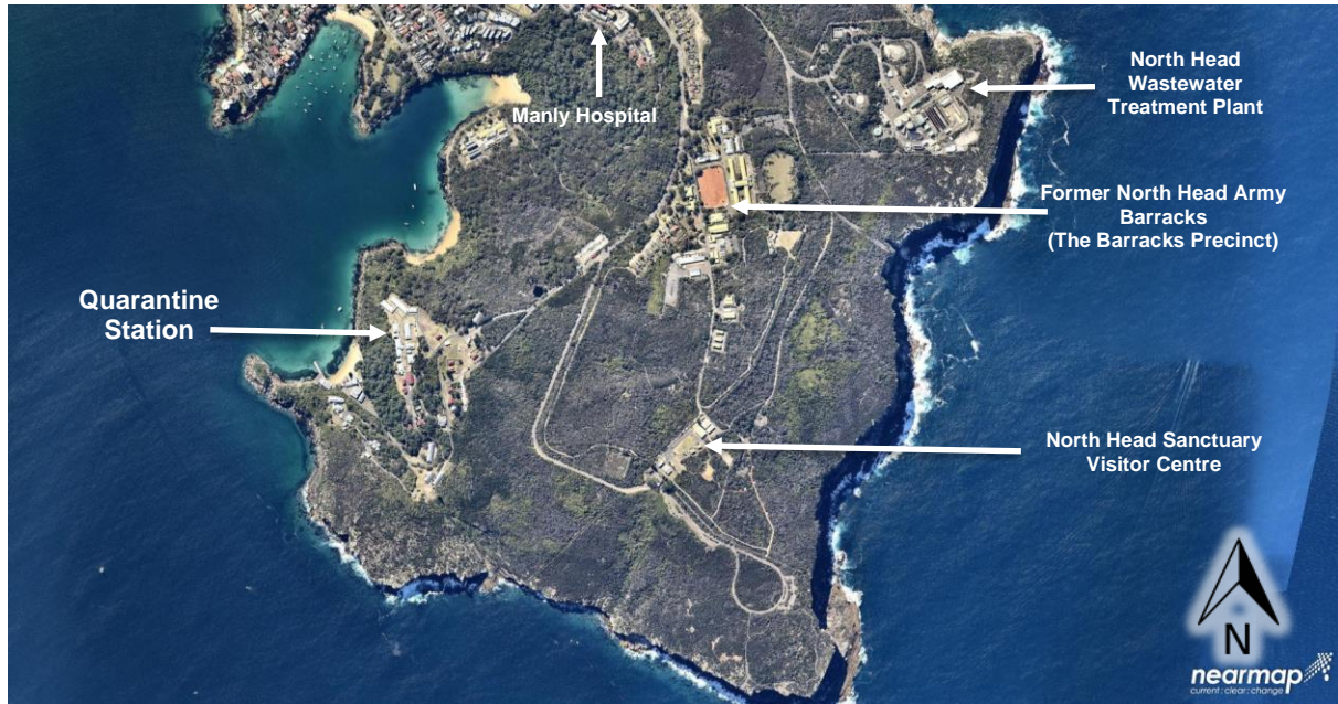
Figure 2: Site Context (Source: NearMap, 2017)
