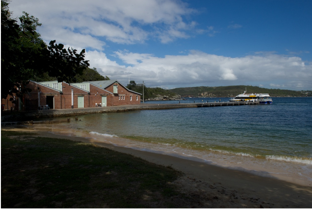
View from beach to wharf, this is the reverse view to those following.
