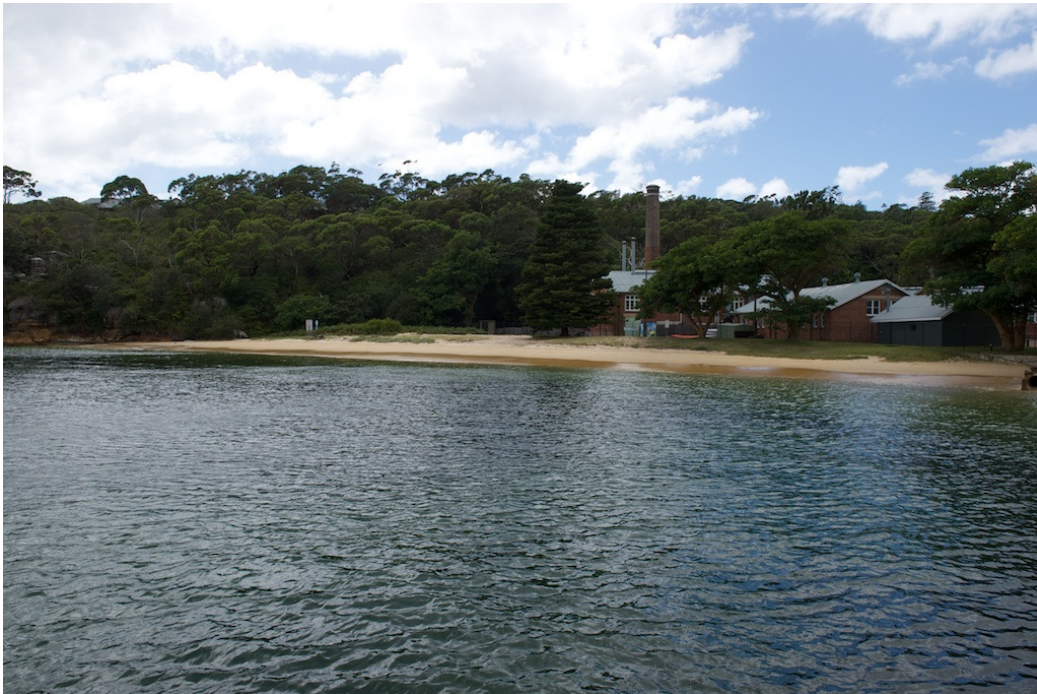
A view from the join between concrete and timber wharf sections. There is no view of the area from this location.
