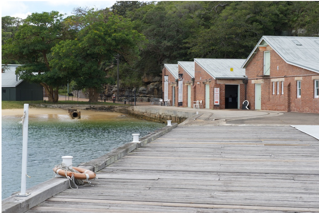
Picture 5: View from the wharf to Building A14-16 (Credit: Paul Davies)
